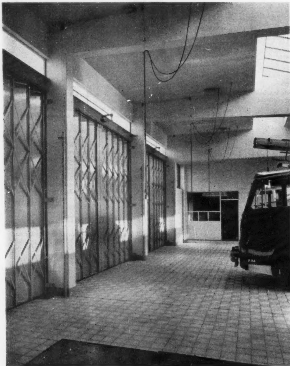
Another view of the appliance room with the watch-room in the background. Sliding folding shutters close the entrance to South Road
