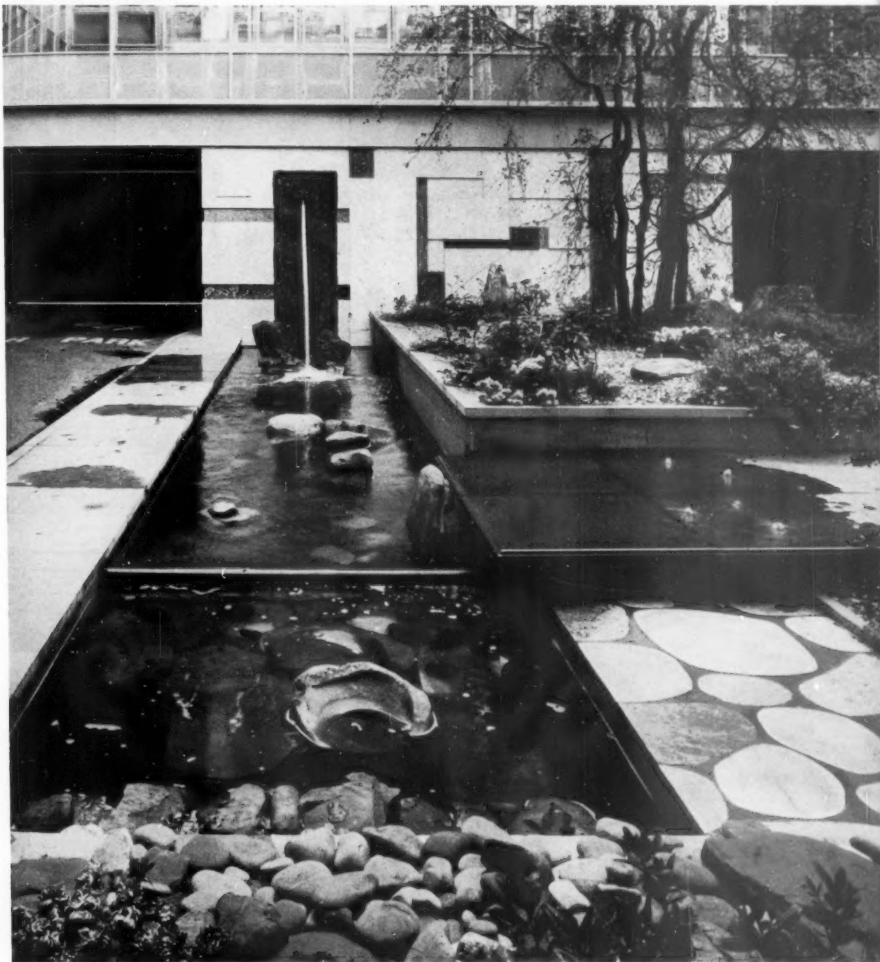
This water garden in the courtyard of a London showroom is interesting for its use of finishes. Note the lining of the pool with stone slabs laid in screed on asphalt and the insertion of a weir to give permanent sparkle.
