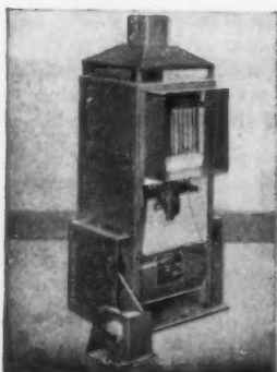
Illustration of Halcyon Model F.43 shown with the ducting removed.
