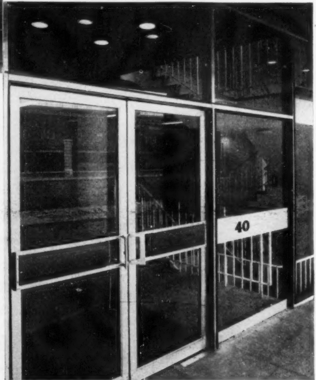
Eastbourne Terrace Development. Architects: C. H. Elsom and Partners. Entrance screens and doors in anodised aluminium with black dyed aluminium beads.
