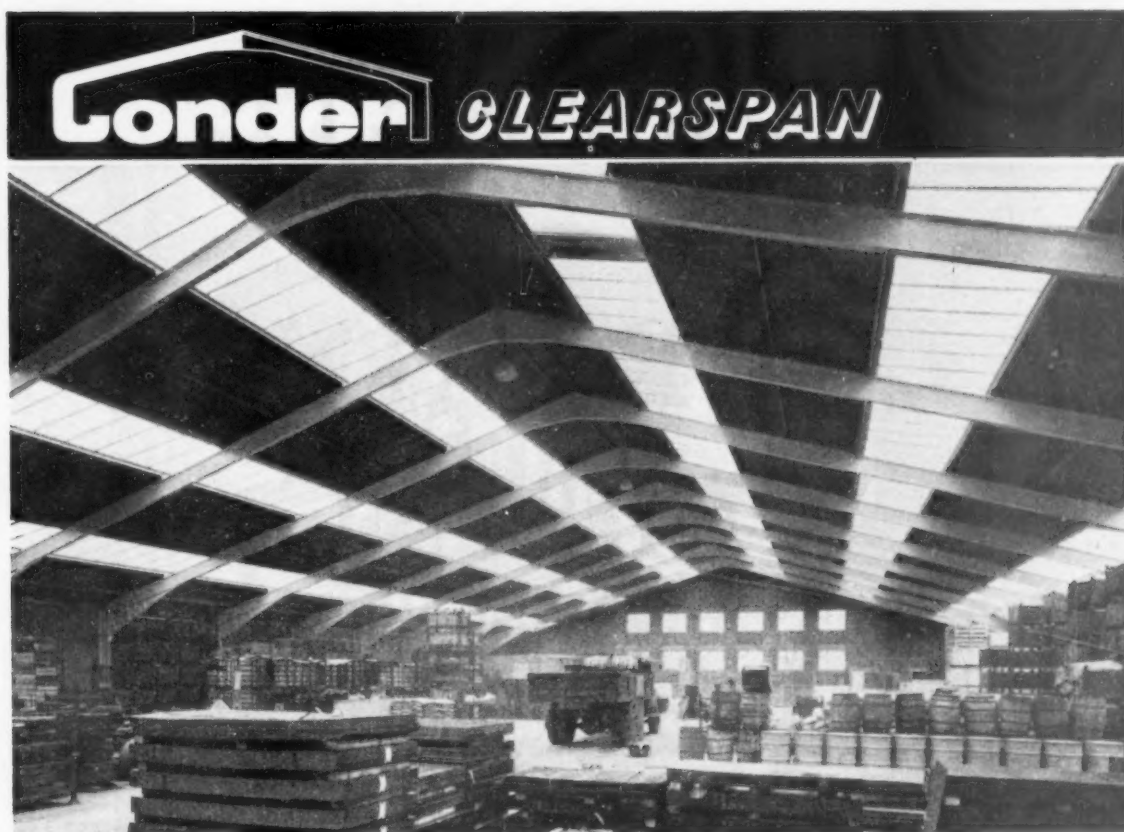
Warehouse, 110ft. span. Gresham & Craven, Ltd., Manchester.
