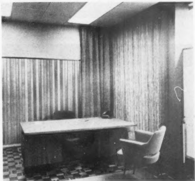
Junior management grade office, showing connection between demountable partitioning and aluminium mullions, centre
