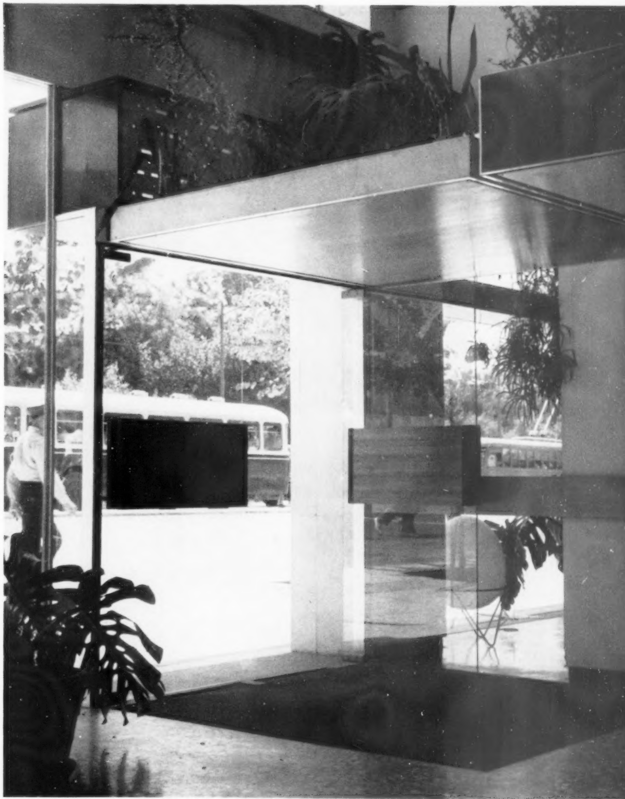
This entrance shows a number of refinements of which the most noteworthy are the coincidence on plan of the canopy and the doormat and enlargement of the door push so that it becomes an architectural plane.
