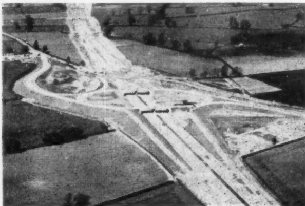
Below, an interchange and service area on the M.1 during construction. The extent of the disturbance shows the need for a comprehensive grading and planting plan
