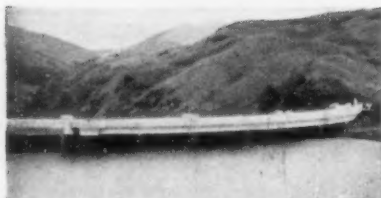
Scotland. THE GLEN SHIRA HYDRO-ELECTRIC SCHEME. Concrete surfaces of the main dam, lower dams, and main tunnel are all FLINTKOTE — protected from attack by acids in the peaty water.
