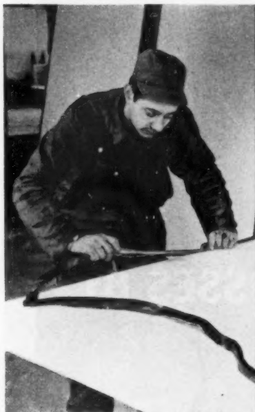
Preformed neoprene gaskets for curtain wall construction are simply installed, seal effectively, outlast conventional glazing compounds. They cut costs and speed construction.
