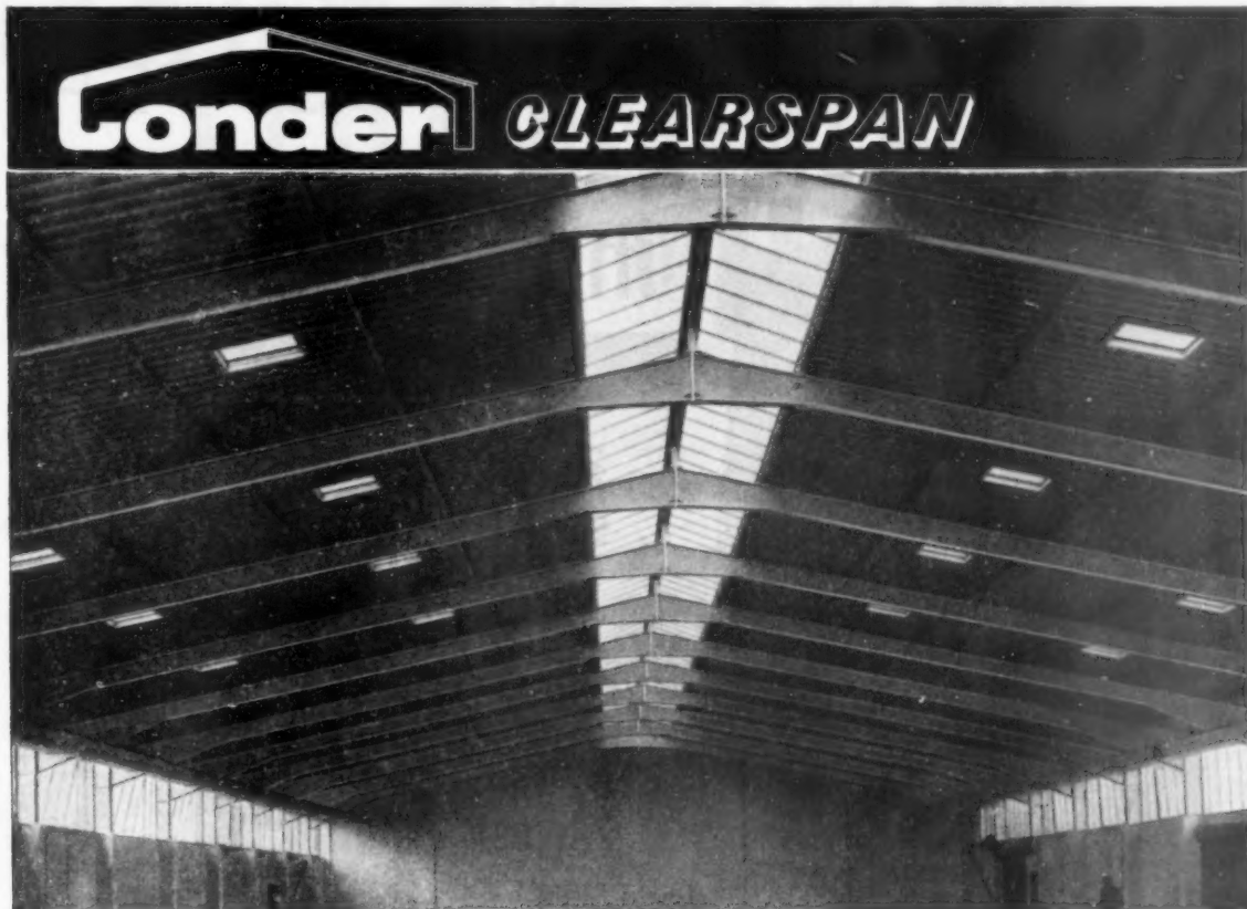
Warehouse, 100 ft. span. Roof Pitch 12°. Alford & Alder (Engineers) Ltd.
