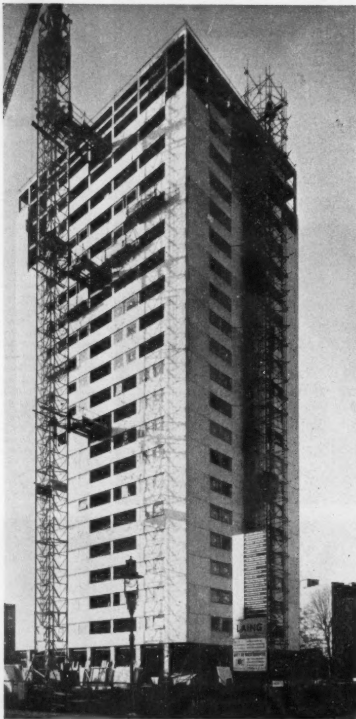
The state of the building on February 8, 1961. The intermediate beams halfway down the top frames are to form viewing slots through the storey height wall of the roof terrace. The general proportions of the finished building can now be assessed.
