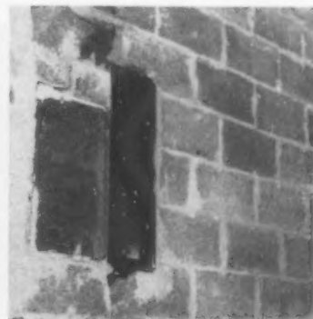
Outside Meter Unit seen from the general circulation area, above. This box contains apparatus which must be accessible to the Electricity Board (see diagram)
