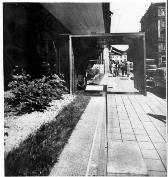
This telephone hood which projects over a public pavement shows a method whereby a public telephone service can be provided on the front of a building with a minimum of visual interruption, At the same time it must be questioned whether the slightness of the projecting parts, when approached from the side, is not a risk to people bumping into the kiosk.
