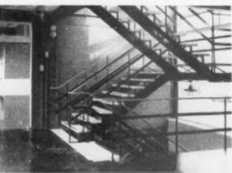
Stairway in laboratory unit. The unclad framing and exposed service runs are typical of this unit
