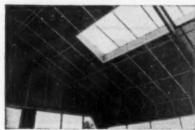
On the left can be seen the great flexibility of the Grecon System, it fits neatly and securely around the existing roof and window lights, and any panel is easily removed and replaced for inspection purposes.
