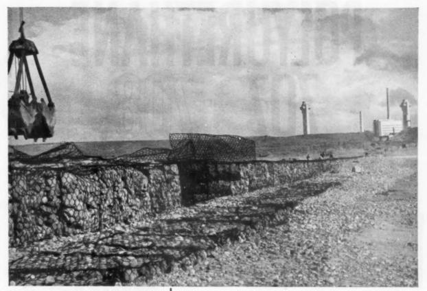
'Gabion' baskets made by Barnards Ltd., Mousehold Works, Norwich, from wire covered with p.v.c. based on 'Corvic' I.C.I. vinyl polymer by Tinsley Wire Industrise Ltd., Sheffield Road, Sheffield 9. They are here being filled with stones and placed in position.
