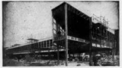
New Air Terminus buildings in Kensington for B.E.A. Photograph taken 16 days after commencement of steel deliveries. Main Contractors : Messrs. Richard Costain Limited. The Architects for the Bowater Paper Corporation Limited's new Office Blocks at both Northfleet and Mersey required Lattice Steelwork on a 3ft. 4in. module. This allowed complete flexibility of internal arrangements and all service lines are easily run between floor and ceiling.
