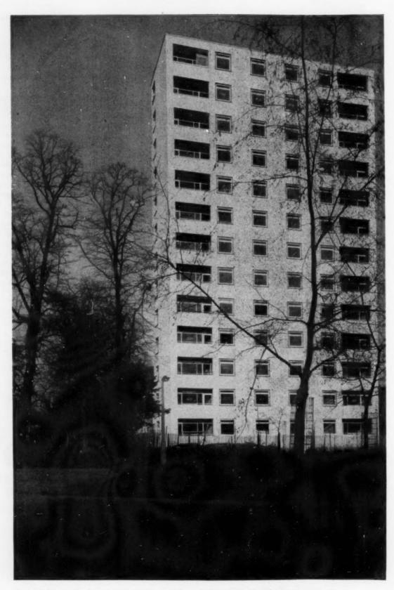
The LCC flats at Wandsworth constructed in unreinforced load-bearing lightweight aggregate concrete
