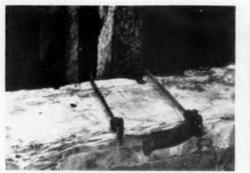
Left: Wire clips for securing shutter to ladder Right: Timber wedge driven through projecting buckle
