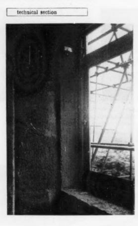
Window frames are secured in position by galvanised straps nailed direct into the concrete
