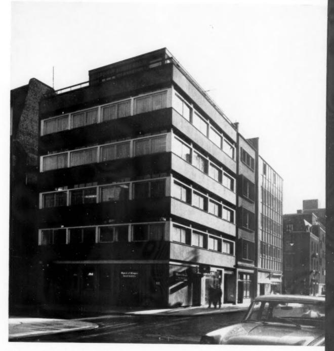
This is an interesting solution to the problem of providing the effect of continuous glazing in a load-bearing facade. The panels below the sill are of in-situ concrete faced with Hornton stone; but the 9 in. by 9 in. concrete mullions (as also the transoms) are faced in 12-gauge pressed aluminium.
