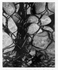
A close-up of one of the 'Gabion' baskets showing the wire coated with p.v.c. based on 'Corvic' I.C.I. vinyl polymer.
