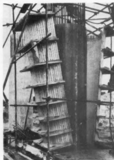
Shuttering lined with Lustrex polystyrene
