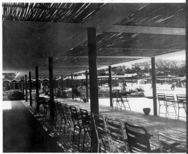
This pergola shows an interesting method of obtaining an even, small mesh pattern of light and shade. Note the careful detailing of the bamboo panels to prevent sagging.
