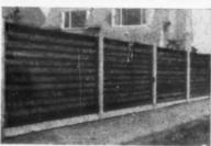
No other type of fence is as strong and rable. The panels are pressure creosot timber and posts of granite concrete. ALL CONDITIONS PROVIDED FOR
