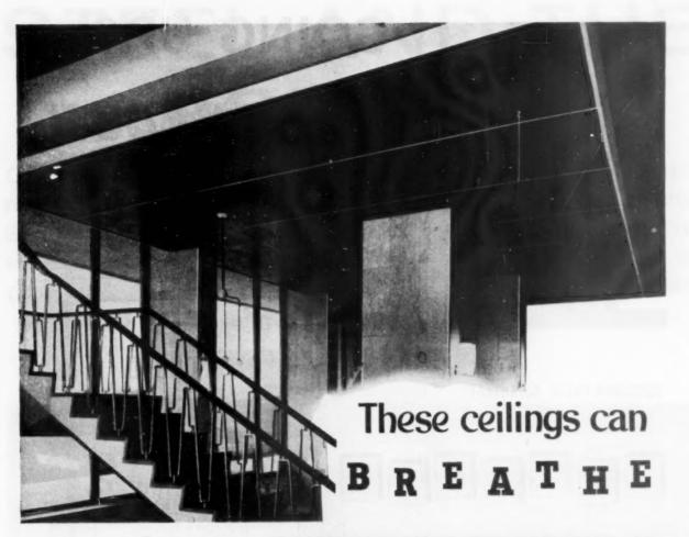
Overhead services are completely obscured, yet there is adequate circulation of warm air *through* the panels to maintain efficient heating.
