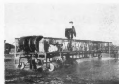
FEB concrete curing spray, below
