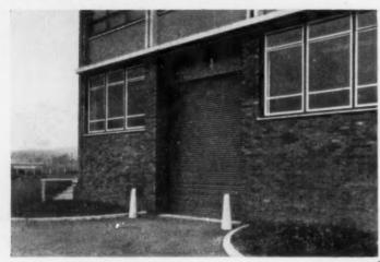
One of the 6 electrically operated Rolling Shutters installed at the new Sandoz Products Ltd., chemical building, Calverley Lane, Horsforth, Nr. Leeds.
