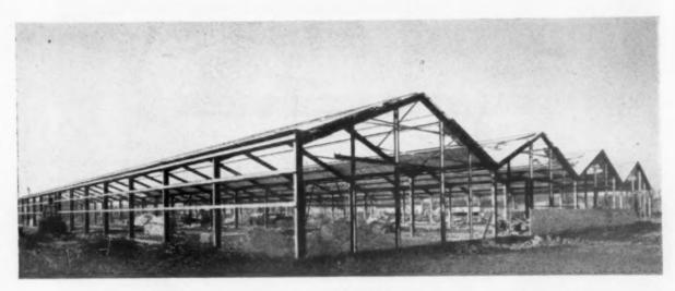
New factory at Daventry comprising four bays each ft. span and 360 ft. long of welded portal frame construction.
