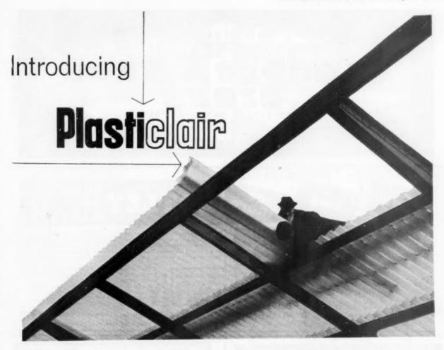
The labour saving modern method of roofing and partitioning Manufactured in continuous length (up to 200 ft.), without welding, PLASTICLAIR makes installations simple and speedy with conventional methods of fixing—less structural support required and long maintenance free life. PLASTICLAIR overcomes the monotony of dull uninteresting surfaces and permits unlimited scope in design, giving daylight advantage.
