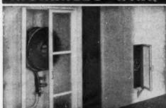
This extremely comprehensive fire protection scheme provides "Safeguard" Hose Reels (fitted in cavities) for use by the occupier and Dry Riser and Foam Inlet Equipment for use by the Fire Brigade.
