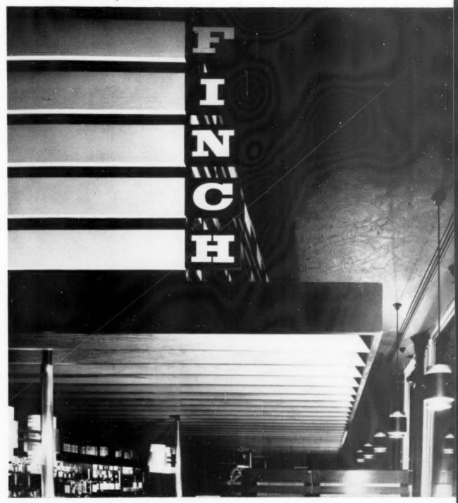
This suspended ceiling is composed of an upper part made of plywood on a m.s. angle frame which, in turn, rests on a "raft" of Parana pine slats. Note the method of supporting the raft on m.s. posts which penetrate the raft visually and are secured to a m.s. flat above the plywood ceiling.
