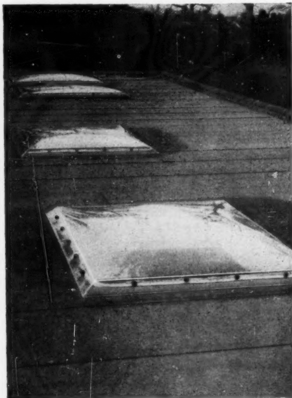
Some of the 94" x 70" Mark II Coxdomes installed over the Weighing-in Room at Lingfield Racecourse, Surrey, for the Racecourse Betting Control Board. Main Contractors, Messrs. Hoad and Taylor Ltd.
