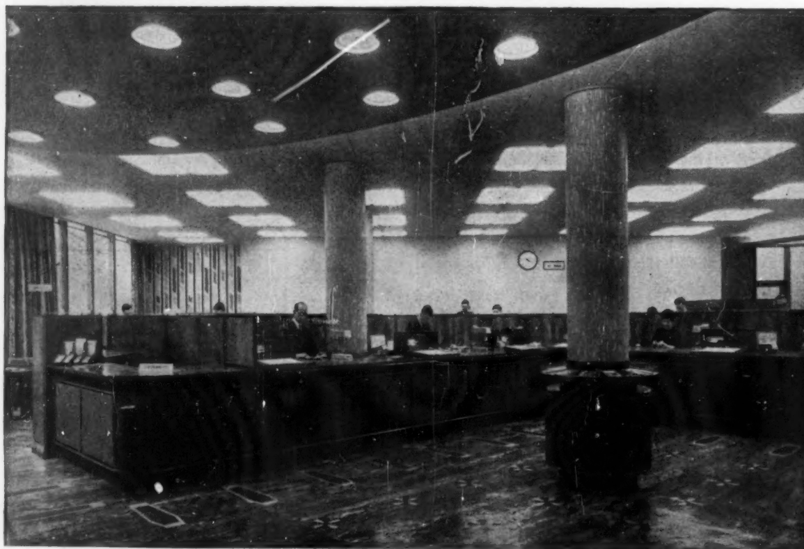
Modular ceiling lighting fittings with opal 'Perspex' diffusing panels made by The General Electric Company Limited, installed in the Midland Bank Ltd., High Holborn.
