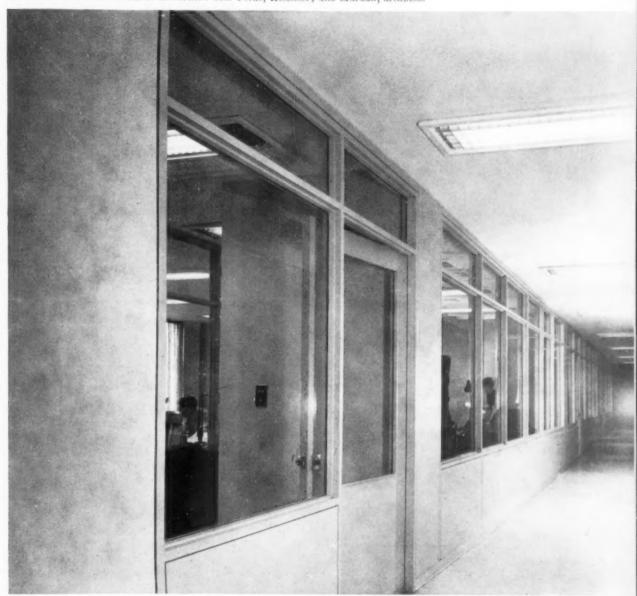
This glazed partition is characterized by its neat detailing at the junctions between its timber framing and the breeze block partition wall.
