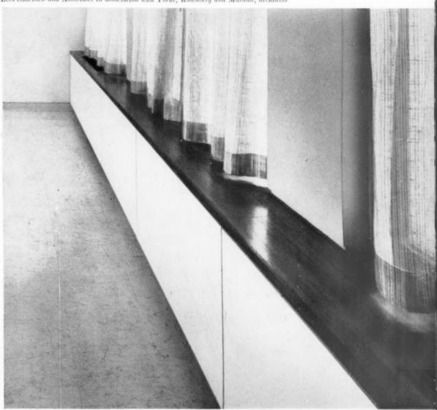
This detail shows a neat method of securing panels beneath an internal sill to conceal heating units, one of which is placed in every second bay with a removable panel in front. Outlet grilles are in the sill.
