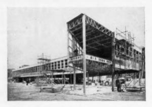
**B.E.A.** For this B.E.A. Building, speed was the essence of the Contract. Sommerfelds designed the Steelwork and from unloading the first lorry on site to the completion of a 250 ton steelwork erection took three weeks.
