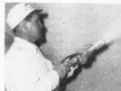
The container from which the Swedish plaster, used as a trial in one of the flats, is forced into the spray gun. In the background may be seen the windows which have been masked with polythene, left
