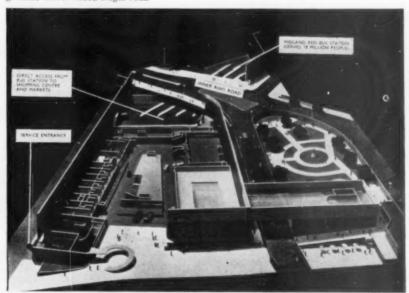
Above, model of the scheme with the lid off, showing circulation system for traffic. The covered shopping area is entirely for pedestrians. Below, view of the covered shopping area, the two levels linked by escalators
