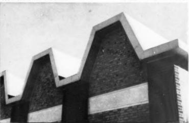
This was achieved by the introduction of timber spacers below the oversailing roof deck units, to which the aluminium soffit was fixed, and the provision of an aluminium angle to bridge the gap between decking and soffit at the oversail line to waterproof the detail and to provide backing for the aluminium fascia.
