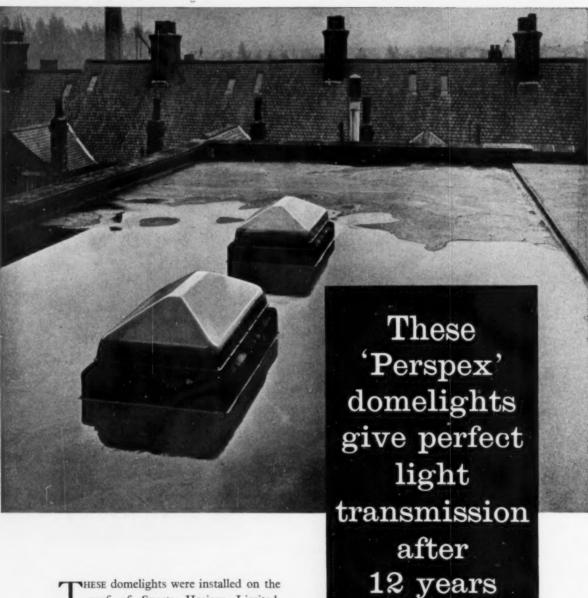
THESE domelights were installed on the roof of Sports Hosiery Limited, Leicester in 1948. As the top photograph (taken in March 1960) shows, weather and the city atmosphere have not affected them at all. They still maintain their high light transmission—a characteristic of 'Perspex' acrylic sheet, from which they were made.
