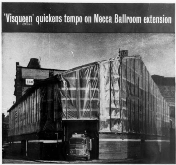
A temporary weatherproof structure clad with 'Visqueen' polythene building sheet over extensions to the Locarno Ballroom, Liverpool, for Mecca Ltd. Contractors: James Crosby & Sons Ltd.
