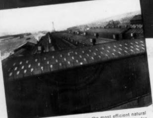
Robertson Round Ventilators are the most efficient natural ventilators in the world. Guaranteed exhaust capacities under varying conditions of temperature difference and wind speed.
