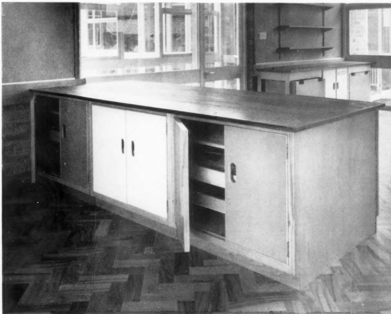
This back-to-back storage unit is framed in beech with plywood-faced doors and end panels. The top is polished iroko and the doors are painted.
