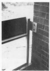
The timber balcony and gallery fronts were fabricated in the joinery shop and fixed to brickwork by galvanised angles which allow good tolerance. A similar front is used for balconies, galleries and service yard screens.
