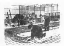
Polythene film damp and soil proof membranes under concrete,
