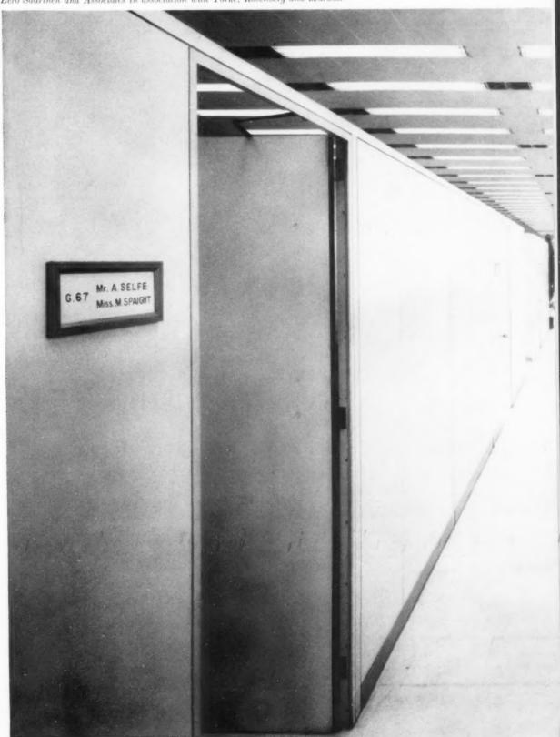
This modular partition (on a module of 5 ft.  $5\frac{11}{10}$  in.) is of standard 2-in, thickness throughout despite the fact that in some positions it carries up to full ceiling height. Note the "flash gap" jointing and the exceptionally neat detailing of door frames,
