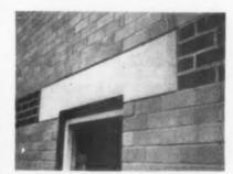
View showing the structural chimney stack supporting reinforced concrete beams, onto which the floors span.
