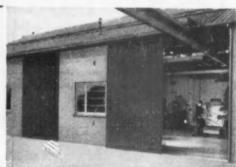
Ellard 'ROLLS' straight sliding and folding door gear is designed for use with both internal and external doors and partitions. A range of sizes for doors weighing from 2 cwt. to 40 cwt. per leaf is available. Barbour Index No. 230
