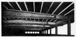
LONG SPAN BEAM CONSTRUCTION 40 ft. and upwards. 4° Pitch.
