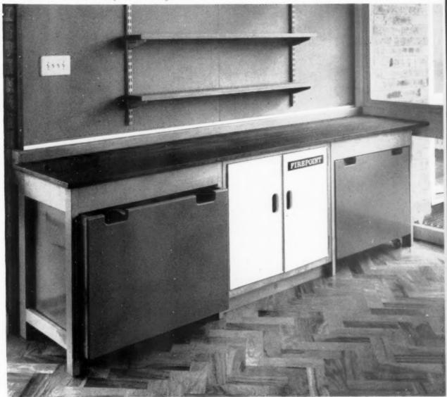
These units (which, like the others in this series, have been tested for some years in use) show that it is possible to design wheeled furniture to roll into spaces with almost as little tolerance round the edges as would be allowed for drawers on runners.
