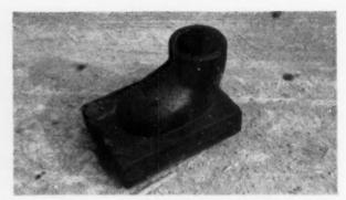
The roofs of the outhouse are drained through an outlet which is a glazed stoneware block-trap, its normal use is for sewer drainage.
