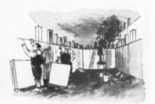
Concrete shuttering made from 'Flovic' vinyl copolymer foil.
