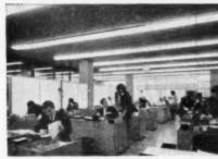
The DAEMPA ceilings throughout Castrol House are fitted with continuous trough cold cathode lighting with diffusers made from diamond pattern 'Perspex' acrylic sheet by Ionlite Limited, Scrubs Lane, London, N.W.10.
