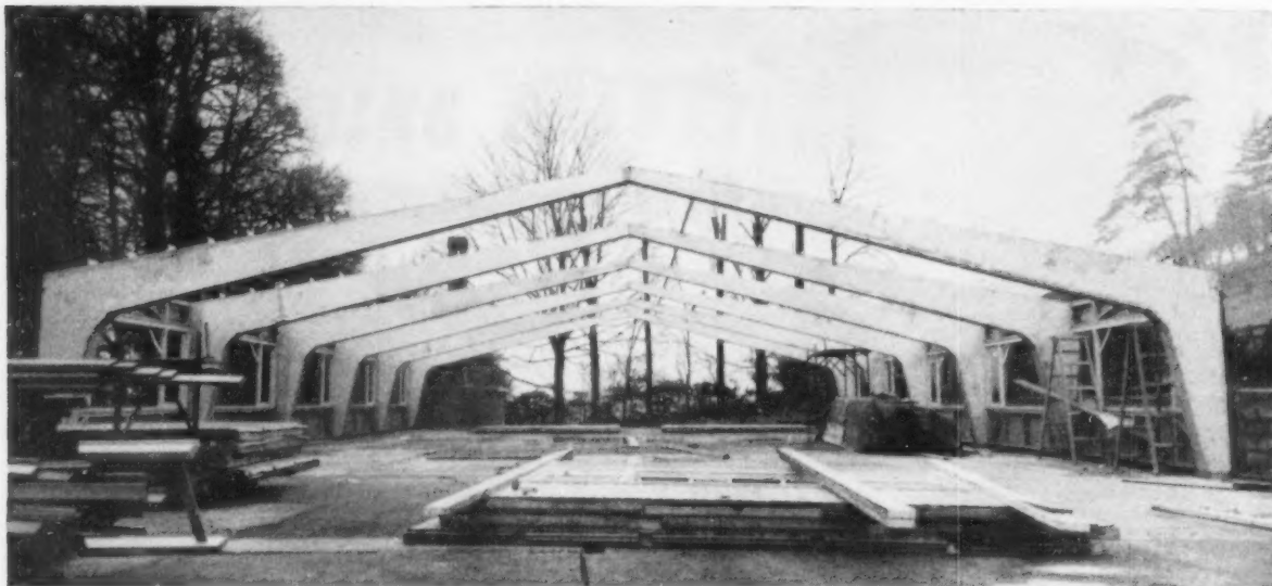
Fifty-nine ft. plywood web portals for offices of Salem Engineering Co. Ltd., Milford, Derbyshire. Designed by D. W. Cooper, B.Sc., A.M.I.Struct.E., F.Inst.W.Sc. Fabricated by F. and H. Sutcliffe Limited.
