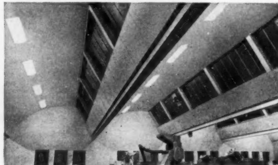
Fluorescent lighting fittings with clear 'Perspex' covers installed in a shell concrete roof structure. Manufactured by A.E.I. Lamp and Lighting Company Limited, Melton Road, Leicester.
