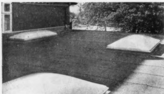
'Duplus' domes made from 'Perspex' acrylic sheet by Duplus Domes Limited, Chatham Street, Leicester, on roof of dining room at Barton Grange Hotel, near Preston. Architect, George H. Broadbent, L.R.I.B.A., A.I.A.A.
