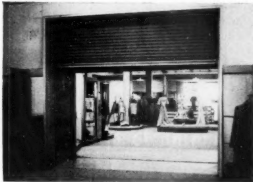
A pair of automatic fire-resisting shutters in a department store.
