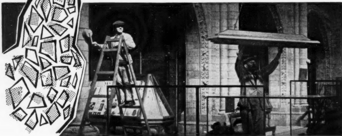
Lights being serviced at the Natural History Museum by means of L.E.F. Raising and Lowering Gear.
