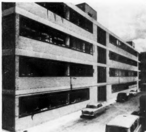
The rear of the factory. The open doors on the balconies, made of steel, are the entrances to the factories. The exposed conduit for the street lamps is due to one of those all-too-easy lapses in the architect's office, but surely this problem could have been solved more neatly by tucking mineral-insulated cable along the top of the floor beam
