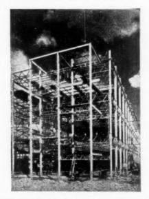
YORK. For the City of York a Grammar School. Sommerfelds designed the Steelwork on a 3 ft. 4 in. modular grid allowing complete freedom for the Architect to use curtain walling and internal arrangements.
