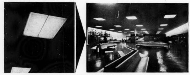
SPECIAL 4' 0" × 4' 0" MODULAR FITTINGS WITH PERSPEX DIFFUSERS USED IN THE BRITISH RAILWAYS TERMINAL AT SOUTHAMPTON. Architect : C. E. Drongoole, A.R.I.B.A. Engineer : J. H. Jellet, O.B.E. M.I.C.E.
