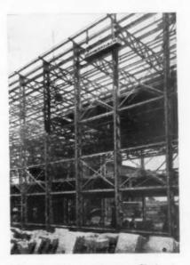
I.C.I. For I.C.I. a Laboratory Block. A multi-storey building with a height to eaves of 44 ft, and uninterrupted spans of 50 ft. on each floor. Deep Lattice Beams and light stanchions were used with considerable saving in steel requirements.
