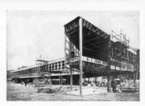
**B.E.A.** For this B.E.A. Building, speed was the essence of the Contract. Sommerfelds designed the Steelwork and from unloading the first lorry on site to the completion of a 250 ton steelwork erection took three weeks.
