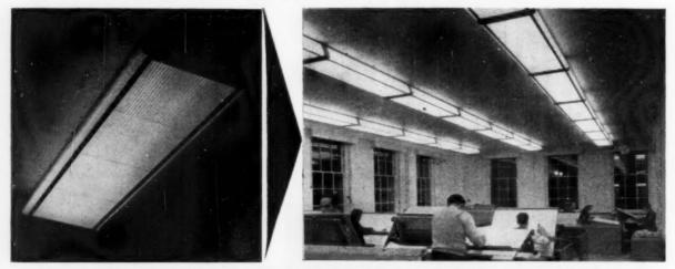
A SPECIAL TWIN LAMP FITTING WITH PARAGRID DIFFUSER AND PERSPEX SIDES MADE FOR THE DRAWING OFFICE OF THE POWER GAS CORPORATION, LONDON.
