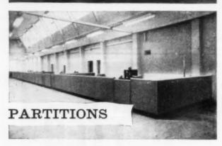
Constructors Metal Partitions are not only extremely pleasing to the eye but of great strength, and serviceability. Their freedom from warping, cracks or decay and their resistance to fire and vermin make them the obvious choice for the sub-division of building interiors. They are very adaptable to changing requirements as they can be dismantled easily and quickly for resiting in new positions in order to use space in the most efficient and economical manner.
