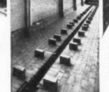
Acid resisting flooring, drain channel and supports for sulphuric and nitric acid pickling tanks. Photograph by courtesy of Garringtons Ltd., Bromsgrave.
