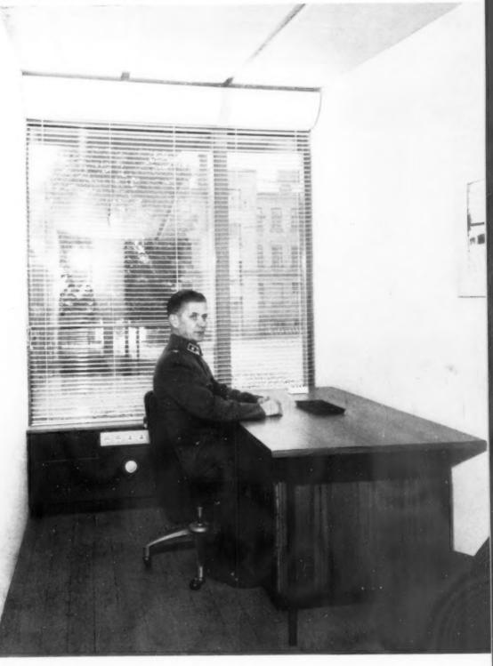
This detail shows the use of an under-sill inlet in a highly insulated air-conditioned building.
