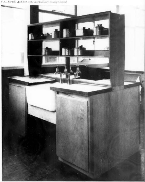
This standard peninsular unit has been developed for housecraft rooms. It is used for the creation of small separate bays and it provides two sinks back to back. The eye level shelves are partly open to assist supervision.
