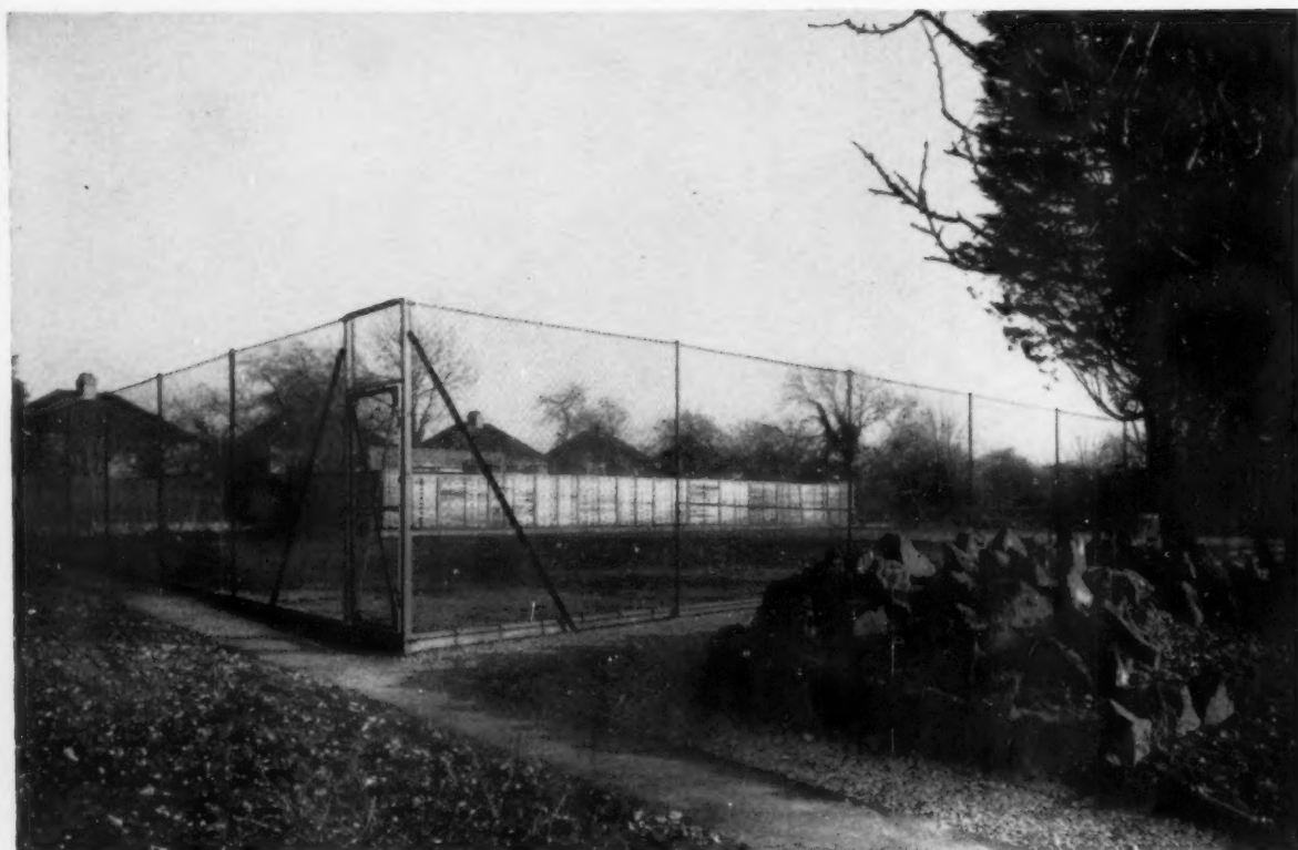
Wire coated with 'Welvic' p.v.c. by Tinsley Wire Industries Ltd., of Sheffield, and made into chain link fencing for tennis court surrounds by Barnards Ltd., Mousehold Works, Norwich. These surrounds were installed for Mr. C. P. Reeve of Bristol by Messrs. H. L. Goodman & Son (Bristol) Ltd., of Temple Way, Bristol 1.
