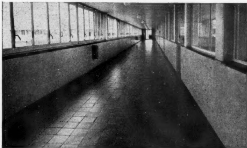
Photographed 19 years after fixing. Corridor at Longton High School, Stoke-on-Trent. Architect: J. R. PIGGOTT, T.D., F.R.I.B.A., Stoke-on-Trent City Architect. Quarry Suppliers: A. WOOD & CO. (Longton) LTD., Tile Fixing Specialists.
