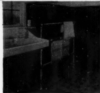
Combined towel airer and radiator keeps the bathroom snug.
