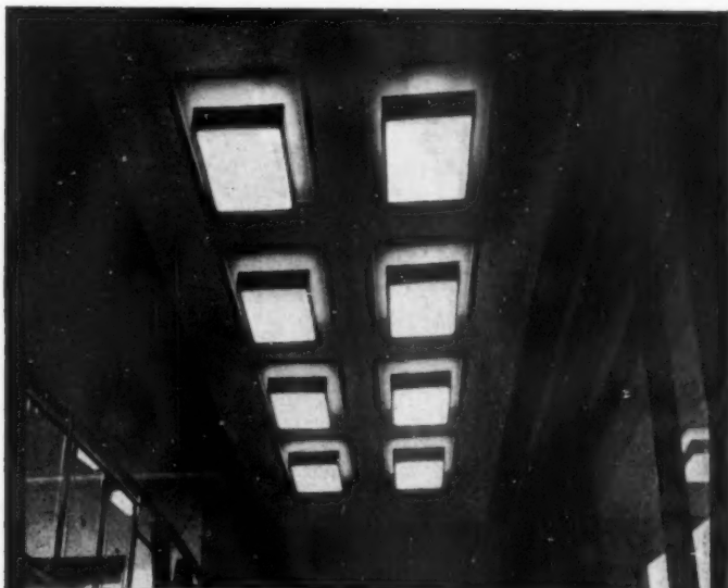
Harris & Sheldon (Electrical) Ltd., designed these special fittings for Woolworth's Head Office. Each houses the three Philips Circular Fluorescent Lamps - 94 watts of fluorescent lighting in a rectangle of small size.
