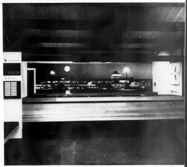
This booking office counter is built up from demountable units. The continuous panel of Parana pine along the front conceals a duct for telephone cables.
