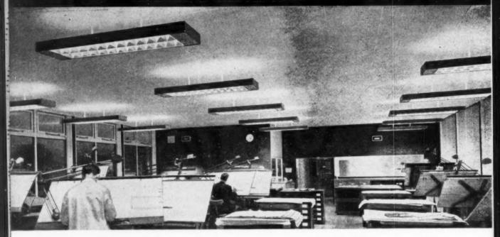
Pleasant working environments with accompanying efficiency call for reasonably high levels of illumination—but such high level illumination must be free from discomfort glare.
