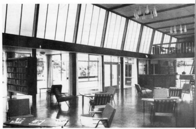
windows, which all come down to floor level. This is a very satisfactory piece of integrated design, which has also largely determined the shape of the building. In order to light the main hall and the reference section, sloping glazing has been used down both sides. This is double-glazed to reduce the heat load, one sheet being non-actinic to prevent overheating in summer. Since all this glazing is fixed, there are four extract fans in the roof.
