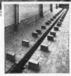
Acid resisting flooring, drain channel and supports for sulphuric and nitric acid pickling tanks. Photograph by courtesy of Garringtons Ltd., Bromserver.
