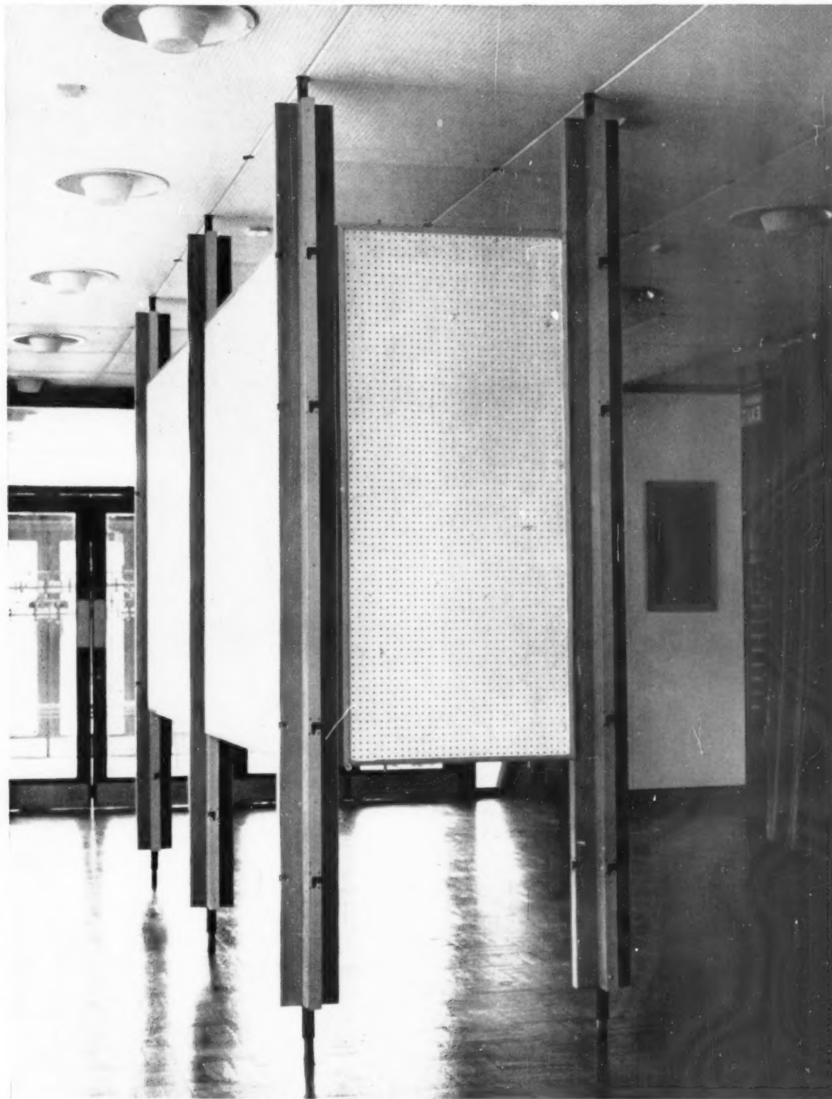
These demountable exhibition screens consist of vertical members on to which various types and sizes of display panel can be erected in different positions.
