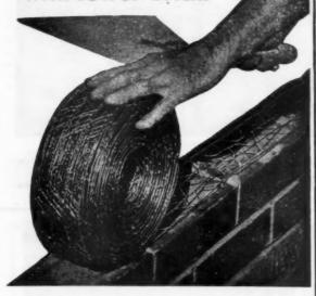
'Bondenn' Reinforcement ends the need for thick, expensive brick walls. 41" brickwork strengthened with 'Bondenn' in many cases replaces ordinary 9" walls. Result - substantial savings in bricks, cement, labour and time.
