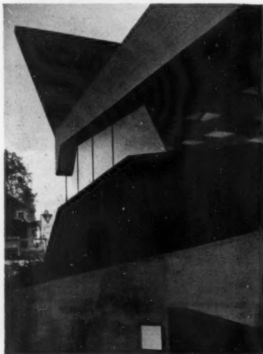
Painted concrete fascia runs round all four sides of the building
