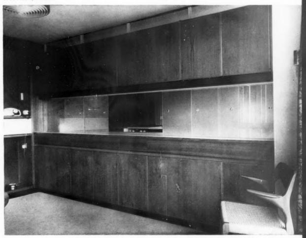
This cabinet, which forms the dividing wall between kitchen and morning room, is an example of high-class joinery work using teak-veneered blockboard and hardwood.
