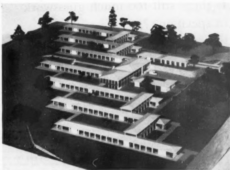
Model of the Horder Arthritis Centre, designed by James Crabtree & Associates, showing low buildings surrounding linked courtyards, with two-storey central treatment, social and administration block. Copper roofs have been chosen, to wear and weather well, and because on the sloping site the roofs will be a dominant feature.
