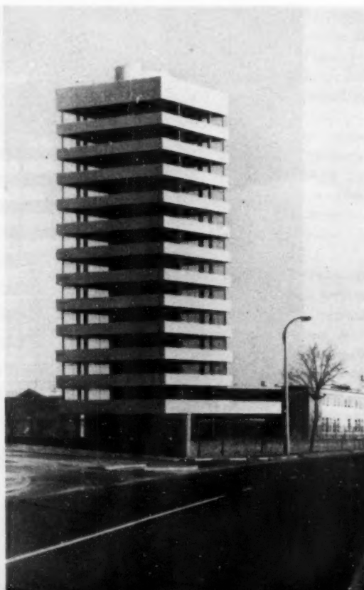
Above, high parapet at roof level, with housing for lift motors and tanks on right. Below, superimposed photograph of the model, showing how closely the original design is in line with the completed building
