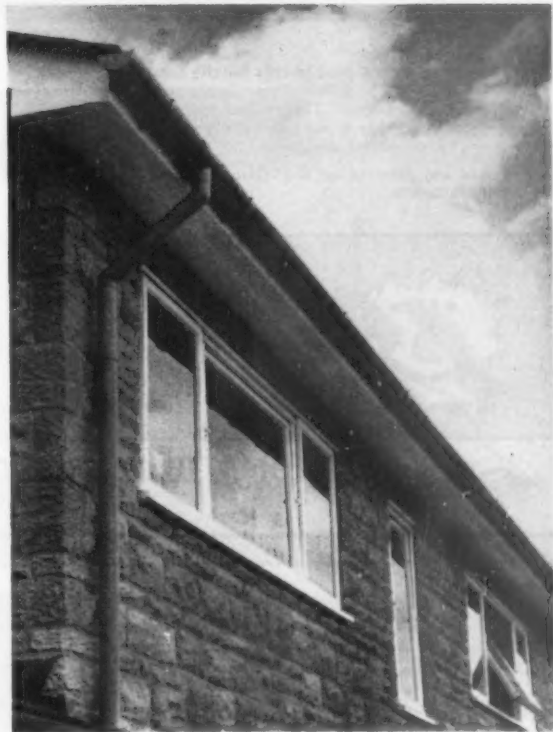
Gutter SNAPS into position on all-weather jointing strip
