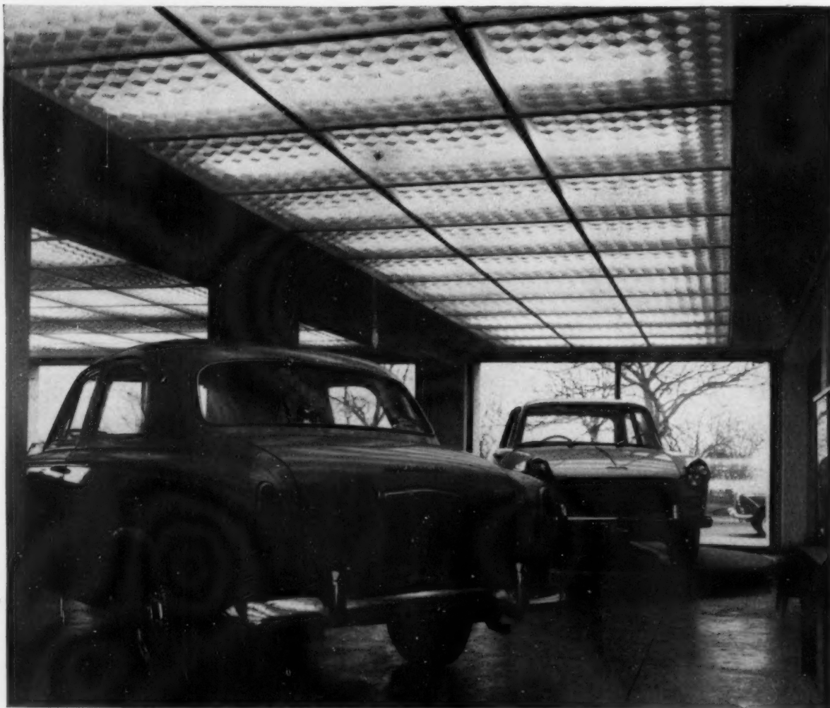
Diffusing panels made from vacuum-formed 'Flovic' by S. C. Errington (Hanwell) Ltd., Uxbridge Road, Hanwell and fitted in a showroom at Messrs. Harold Webb Motors Ltd., London Road, Hadleigh, Essex.
