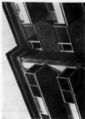
Glass fibre panels on balconies
