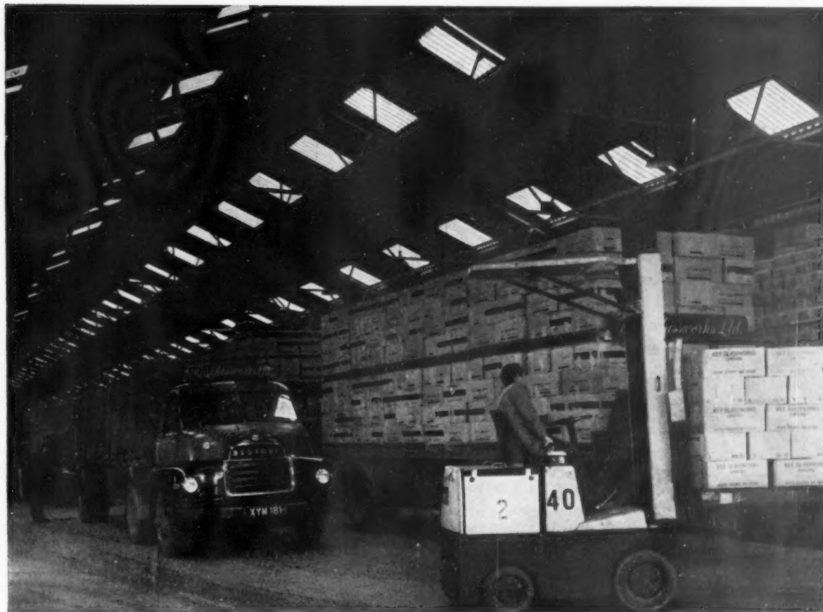
Corrugated 'Perspex' rooflights in a new warehouse at the Key Glassworks Ltd., Edinburgh Way, Harlow, Essex. Architects & Surveyors: Messrs. Brown & Brown, London, N.1. Main Contractors: Messrs. W. & C. French Ltd. Structural Engineers: Messrs. Matthew T. Shaw & Co. Ltd.
