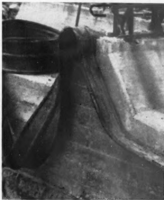
Fig 11 A reservoir expansion joint showing continuity of a bulbous rubber water stop
