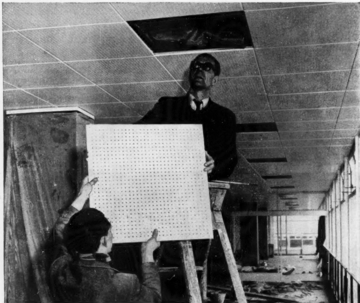
Perforated "Asbestolux" acoustic panels, made by Cape Building Products Ltd., being installed in the ceiling of the 1st floor restaurant in the recently opened International Terminal Building at Birmingham Airport. The backs of these panels were covered with 'Melinex' I.C.I. polyester film on the site to act as a dust barrier. (Below) The finished installation. The panels were installed by the Darlington Insulation Co. Ltd. Main Contractors: Wilson Lovatt & Sons Ltd., Wolverhampton. Architects: Norman & Dawbarn, 7 Portland Place, London, W.1. Photographs by courtesy of Birmingham Corporation.
