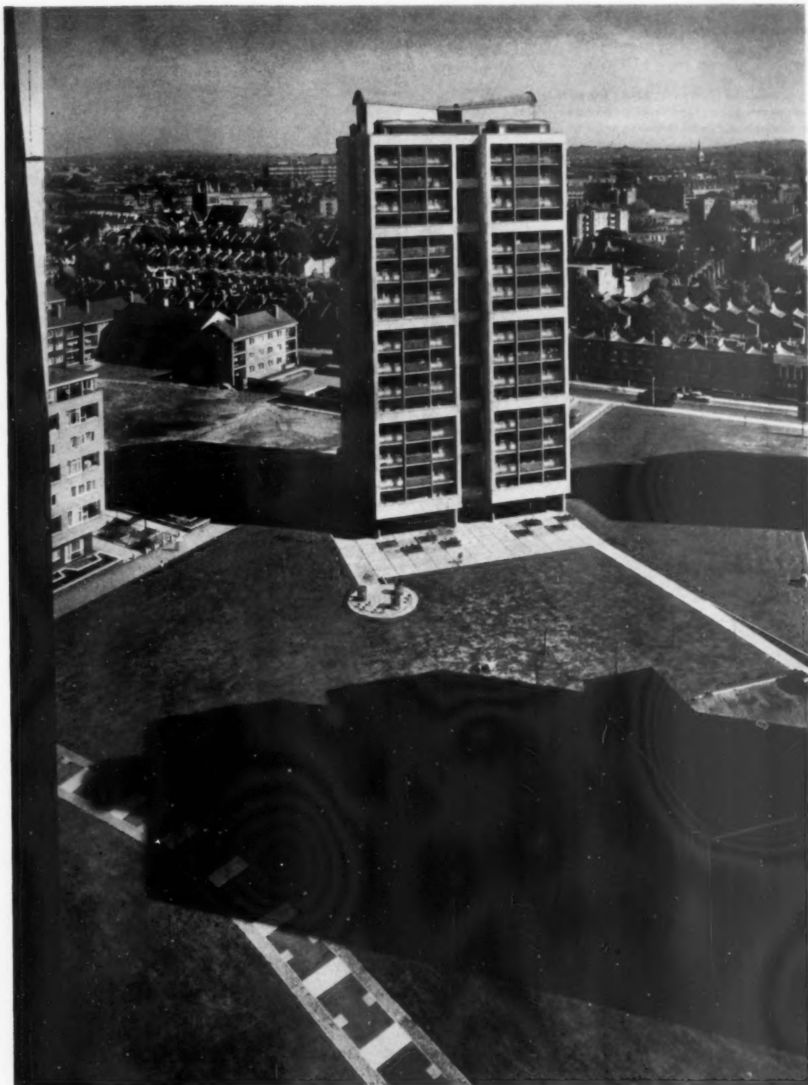
Paths and play areas . . . "conceived as elements in the ground pattern seen from the nearby tall buildings." The deep beams at every fourth floor of the towers, have an important structural function (as well as an obvious aesthetic scale-giving function)—they transfer the loads of the columns they carry out to the flank walls, so that the columns themselves can be kept small, and the whole building supported on a minimum number of pilotis at the ground floor
