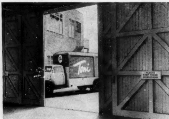
Top hung passing timber doors on Size 4 King Tubular Track—at the garage of Gillette Industries.
