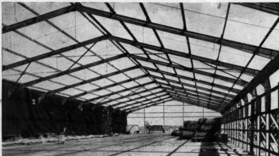
90-ft. Span Rod Processing Building for British Rope Ltd
