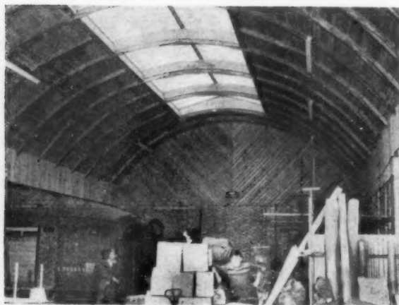
Fig 6 Internal view of timber barrel over British Railways parcels depot at Coventry
