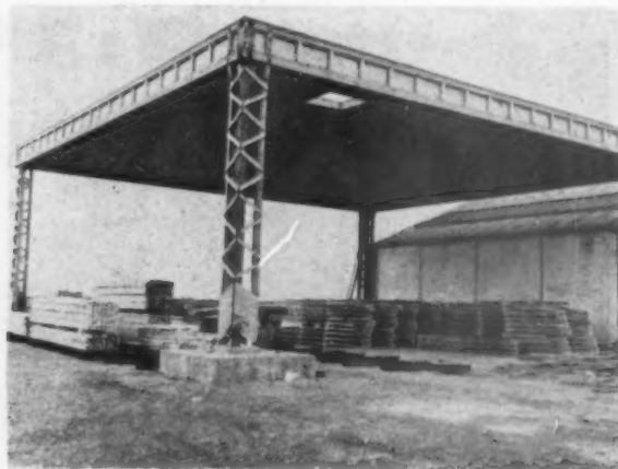
Fig 7 Cross vault over storage shed at Rainham
