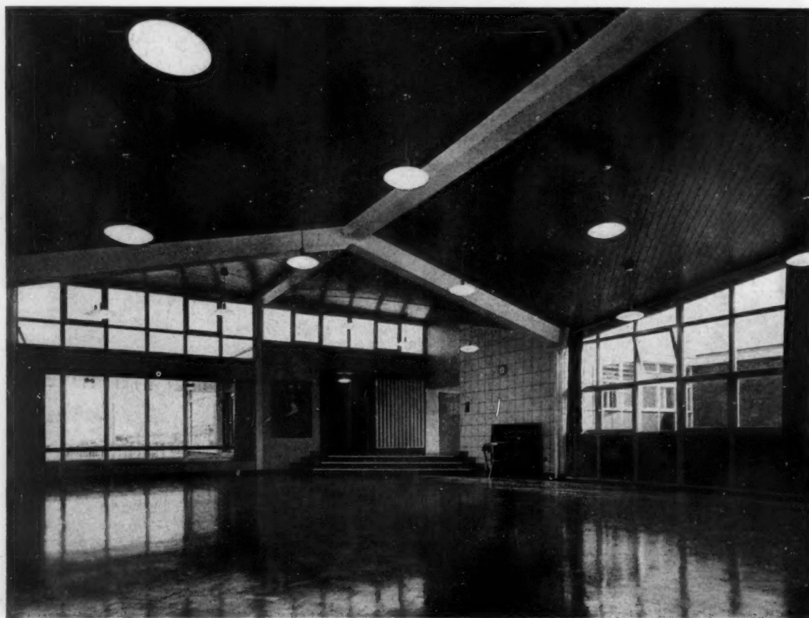
Fig 11 Internal view of hyperbolic paraboloid roof over assembly hall at Wigstone Fields Infants School, Leicester
