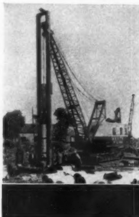
Large mobile piling machine
