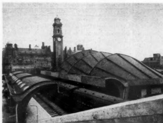
Fig 8 Timber conoids over Oxford Road Station, Manchester
