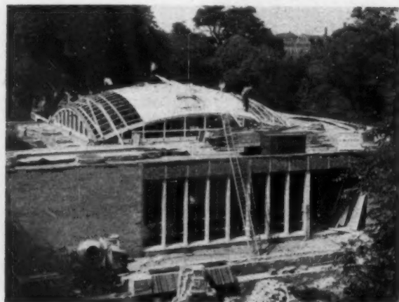
Fig 5 Timber barrel vault at Druntsey School being constructed by schoolboys, right
