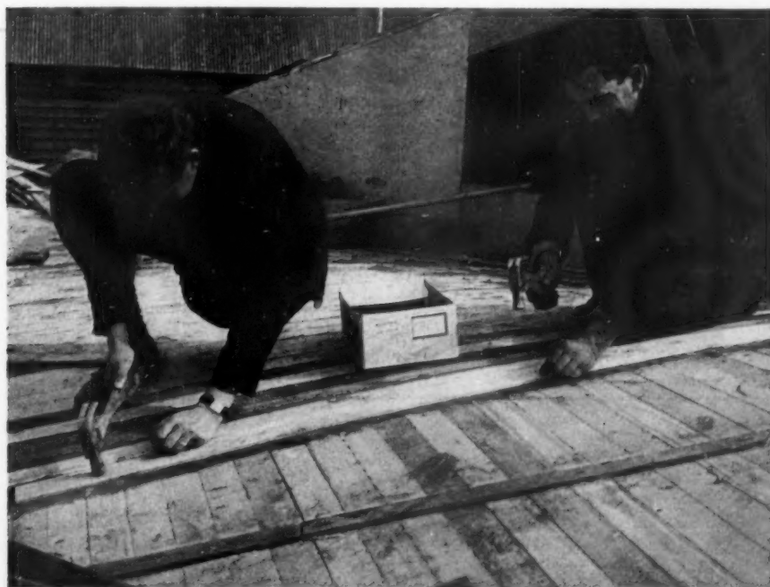
Fig 1 Shell under construction showing the second layer of boards being fixed
