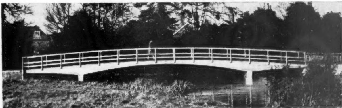
Footbridge at New Sarum, Salisbury, made by Kingston (Architectural Craftsmen) Ltd. The six laminated beams are jointed mid-span to give an overall length of 77ft.
