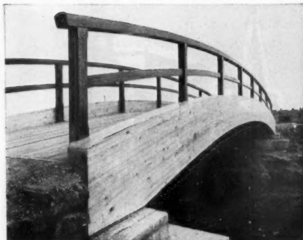
Footbridge, 38 ft span, at Grangemouth, designed by T. Harley Haddow & Partners and made by Muirhead & Sons Ltd.
