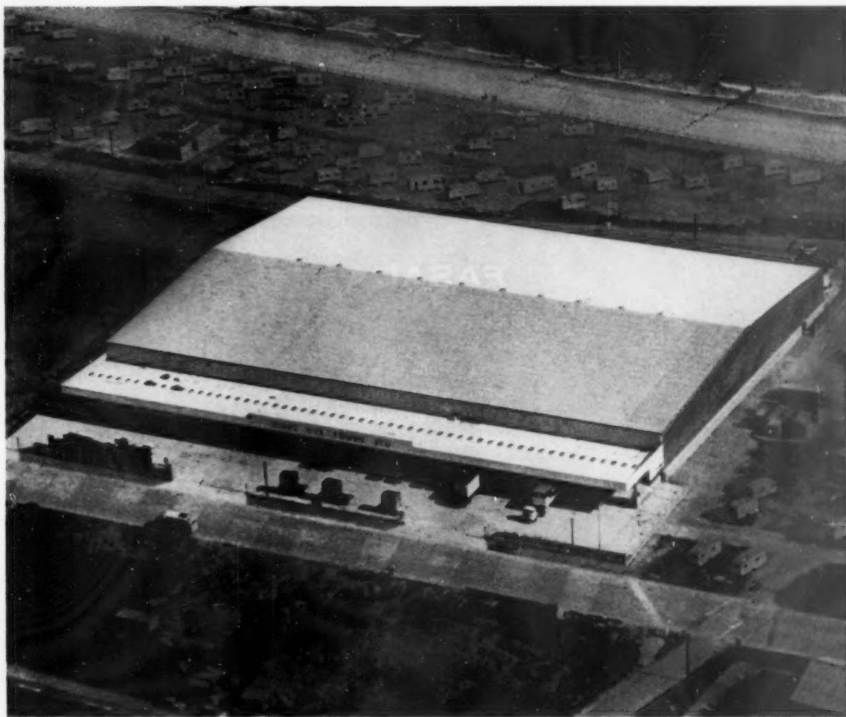
An aerial photograph showing the vast single span roof of the new "Birds Eye" Cold Store at South Denes.
