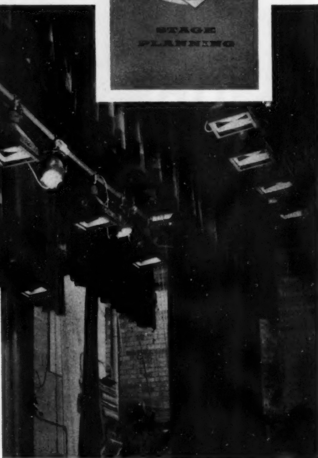
A recent installation at Upper Canada College by Strand Electric Ltd., 36 dimmer circuits controlled by a Strand SR Remote Control board are used. Opposite is a Strand remote control desk for 72 transistor-controlled dimmers.
