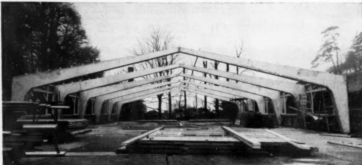
Fifty-nine ft. plywood web portals for offices of Salem Engineering Co. Ltd., Milford, Derbyshire. Designed by D. W. Cooper, B.Sc., A.M.I.Struct.E., F.Inst.W.Sc. Fabricated by F. and H. Sutcliffe Limited.
