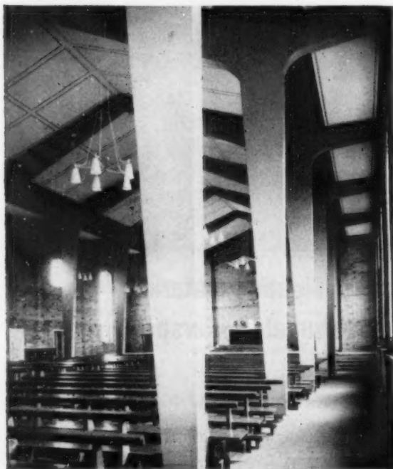
Church of the Sacred Heart, Rochdale, Lancashire. Cantilever arm portals fabricated by F. and H. Sutcliffe Limited.
