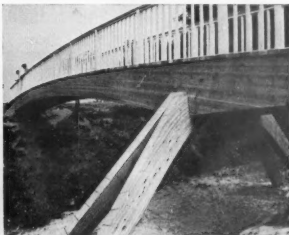
Footbridge at Harlow New Town for the Harlow Urban District Council. Engineer A.W.R. Webb, A.M.I.C.E., M.I.Mun.E., M.R.S.H. The bridge consists of two laminated beams 66ft long giving a clear span of 50ft. The sup- ports are also of laminated construction. The bridge was built by Laminated Wood Ltd, of Bideford. The main con- tractors were Walter Holme & Sons Ltd, Liverpool.
