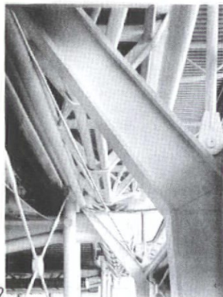
2 Underside of bridge truss showing the braced cradle arms.
