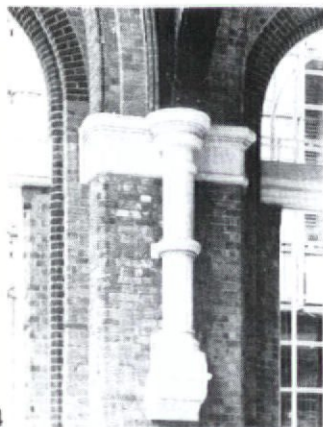
4 Detail of a stone gun barrel bracket which supports the wrought iron spandrel.
