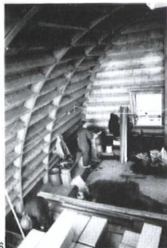
6 The roof under construction. The external plywood cladding is in place, but there are no internal finishes yet.
