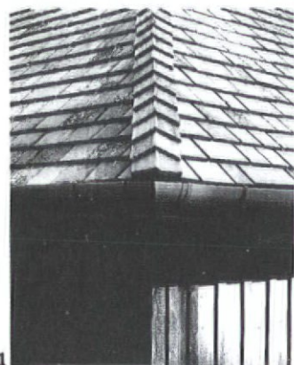
1 Cedar roof shingles are used everywhere except on the main hall, which has a tiled roof. Preformed units are used for the hips. 2 The Heritage Centre is set in a mature Scots pine plantation in Windsor Forest.
