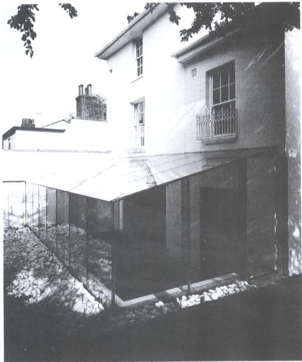
1 The front of the house in Hampstead, north London. 2 The new glass extension, on the north-facing rear of the house. The ground slopes down to the back of the house, so the base of the glazed structure sits on a concrete retaining wall.
