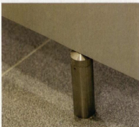
Front cover: cubicle run at Chelsea Village. Above left: the stainless steel leg is out of sight from front view. It is anchor bolted to the floor and a stainless steel pin secures to side panel. It is adjustable on site. Above right: the stainless steel lock is well engineered to ensure a silky-smooth action
