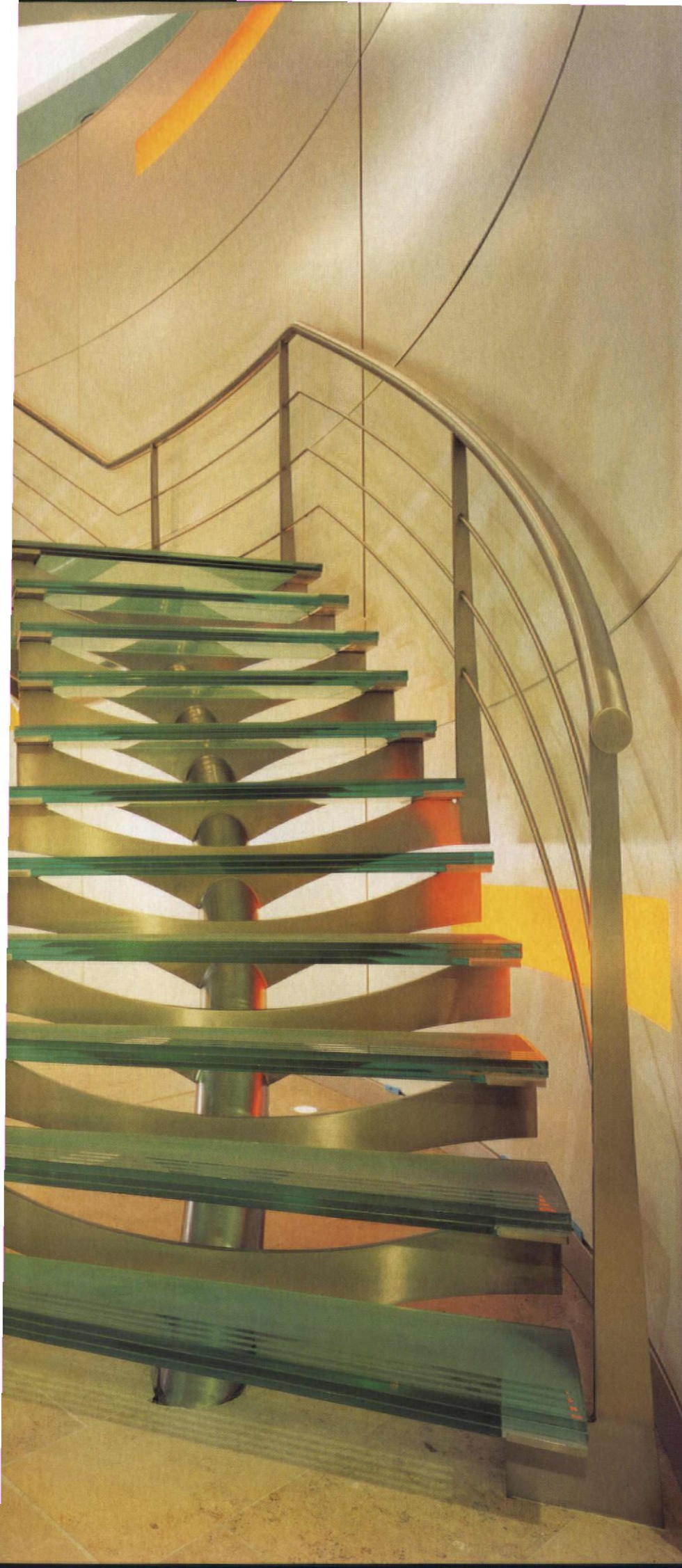
The curved stainless-steel tube has stainless-steel tread supports projecting from it to hold up the toughened and laminated glass treads
