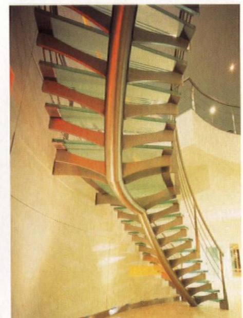
The curved stainless-steel tube has stainless-steel tread supports projecting from it to hold up the toughened and laminated glass treads
