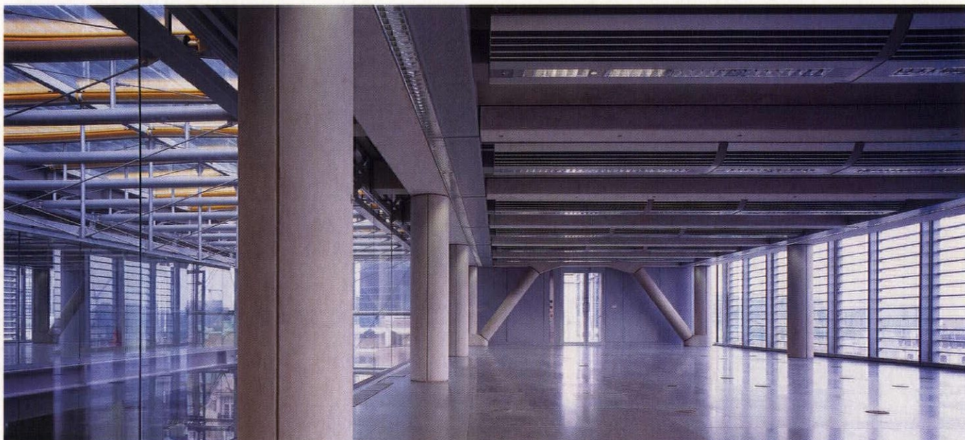
Above: chilled beams give a strong character to workspaces, dispelling the depressing blandness induced by suspended ceilings. Below: naturally ventilated lightweight glazed atria act as climatic buffers, mediating between the external climate and that of the offices
