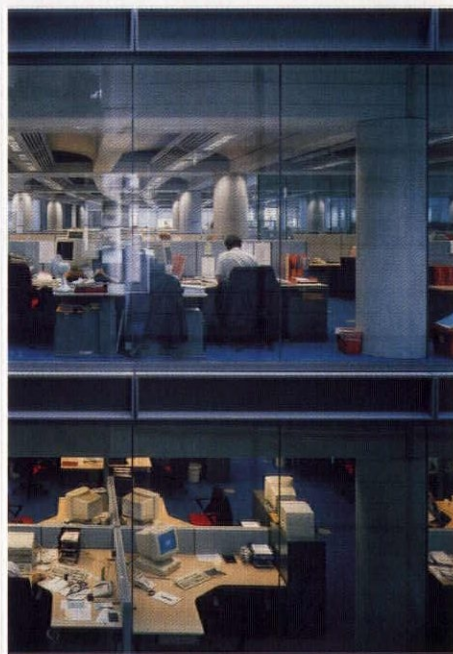
Above: chilled beams give a strong character to workspaces, dispelling the depressing blandness induced by suspended ceilings. Below: naturally ventilated lightweight glazed atria act as climatic buffers, mediating between the external climate and that of the offices
