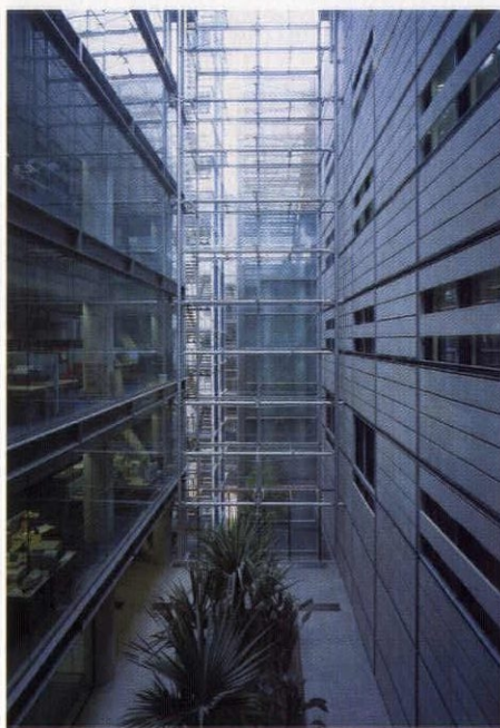
Above: chilled beams give a strong character to workspaces, dispelling the depressing blandness induced by suspended ceilings. Below: naturally ventilated lightweight glazed atria act as climatic buffers, mediating between the external climate and that of the offices
