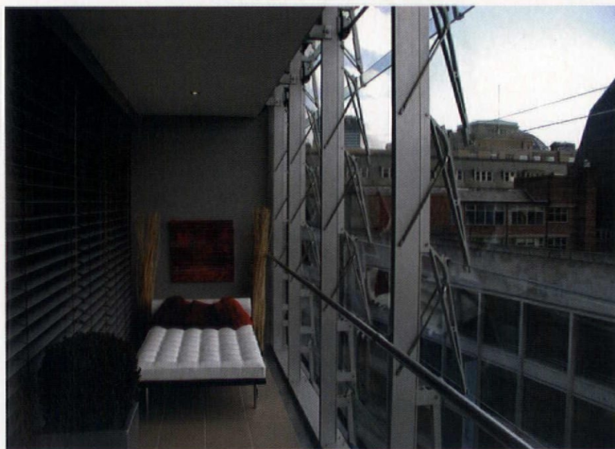
The show flat's 'buffer zone': the louvres close automatically when they detect rain
