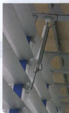
On dull days, light sensors will automatically open the fins to allow maximum vision to the external environment.
