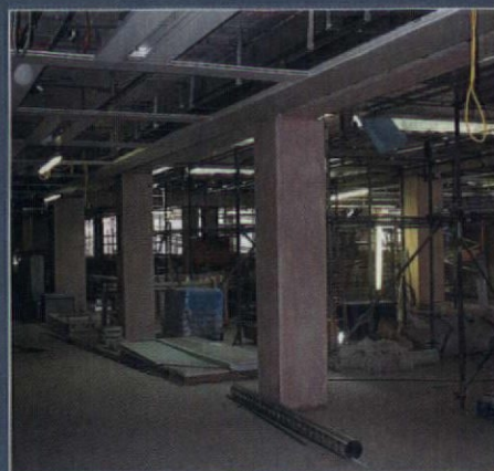
One of the centre-line row of columns, with services squeezed into the ceiling zone
