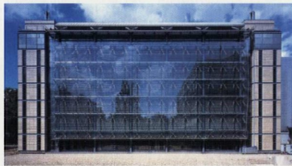
The glazed, solar ventilating facade of the Darwin Centre
