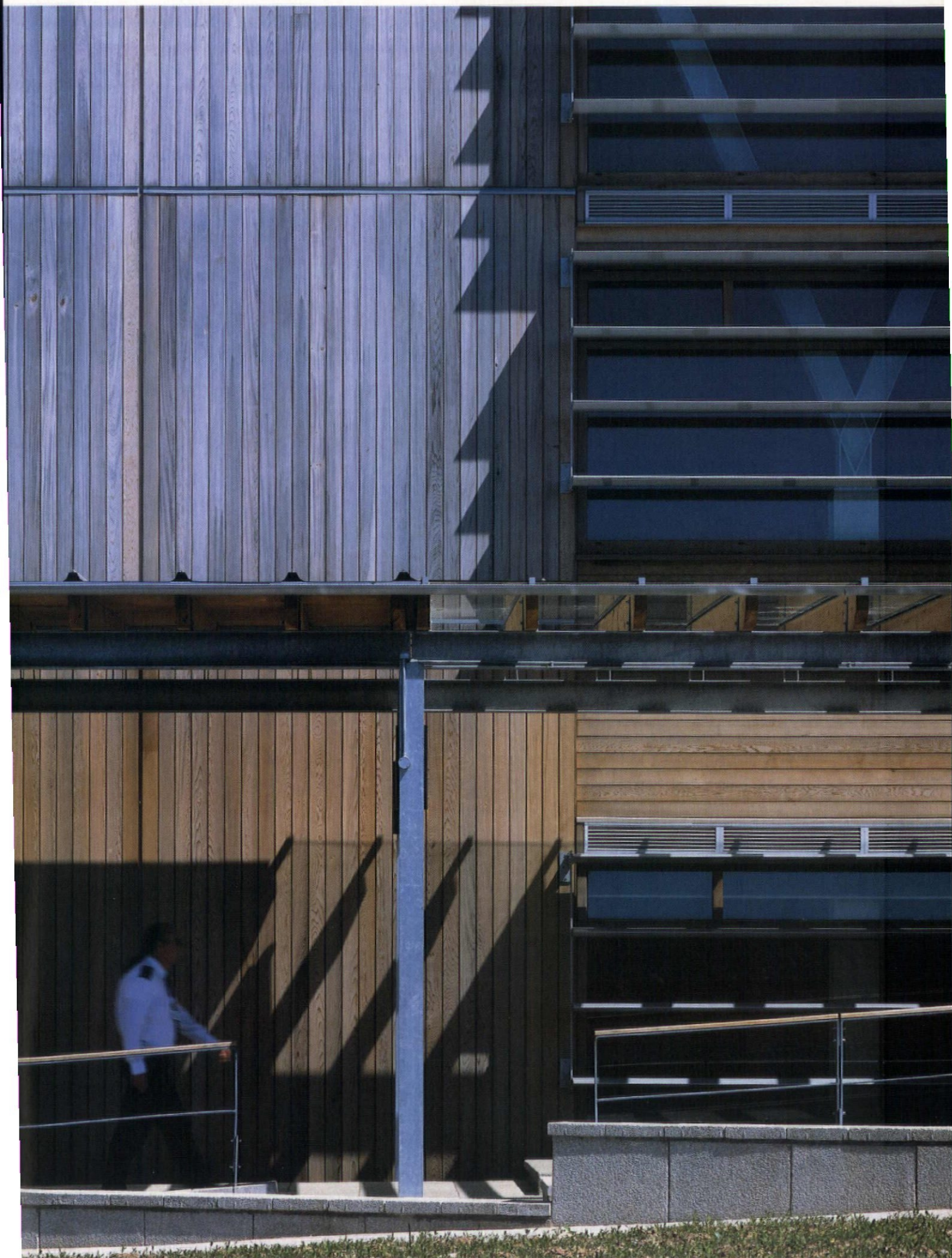
The external timber cladding is untreated and intended to weather – it has already acquired a suitably mellow look
