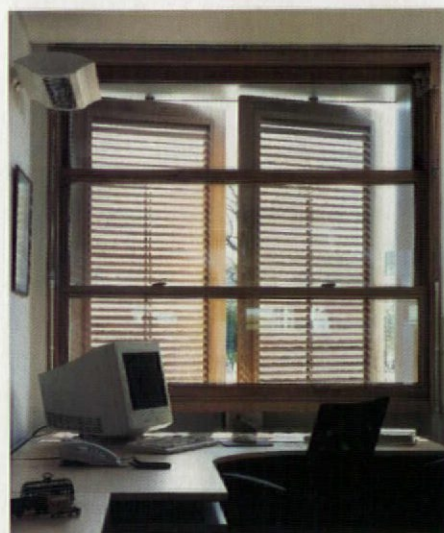
Top: the reception area links the two pavilions. Above: manually controlled windows and shutters
