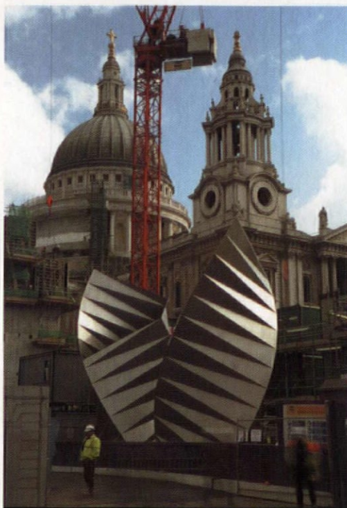
Designer Thomas Heatherwick has unveiled these two 11m-high sculptures in Paternoster Square. The artworks, which have been likened to 'angel's wings', also act as cooling vents for a London Electricity substation. Heatherwick developed the design through experimenting with the repetition of isosceles triangles to form a complex helical form. The 'wings' are constructed from stainless steel which has been blasted with tiny glass beads to create a satin finish. Stanhope and Mitsubishi Estates commissioned the sculpture as a new focus for Bishop's Court, at the western end of the square.
