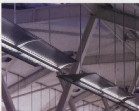
Left to right: light scoops/chimneys extract stale air; 'winged' light fittings act as sound dampers; and louvered shutters control solar gain
