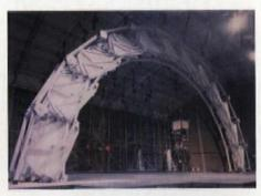
pendent steel arch structure, which also support the loads generated by the guided slots in the outer screen panel. The lowest panels at the base of the arch run along a sliding track which enables the complete system to retract and also partially supports the vertical and horizontal loads.
