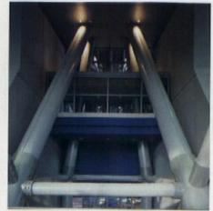
The magnificent folded roof (left) soars over the main space (right) of the Messe. It is buttressed by 12 huge steel A-frames (above) that rise five storeys
