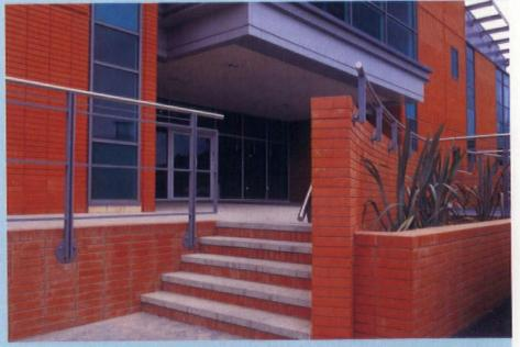
Stack bonding achieves a uniform appearance in brickwork
