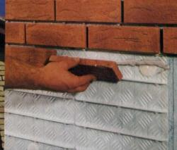
Lightweight prefabricated cladding panels with brick slip
