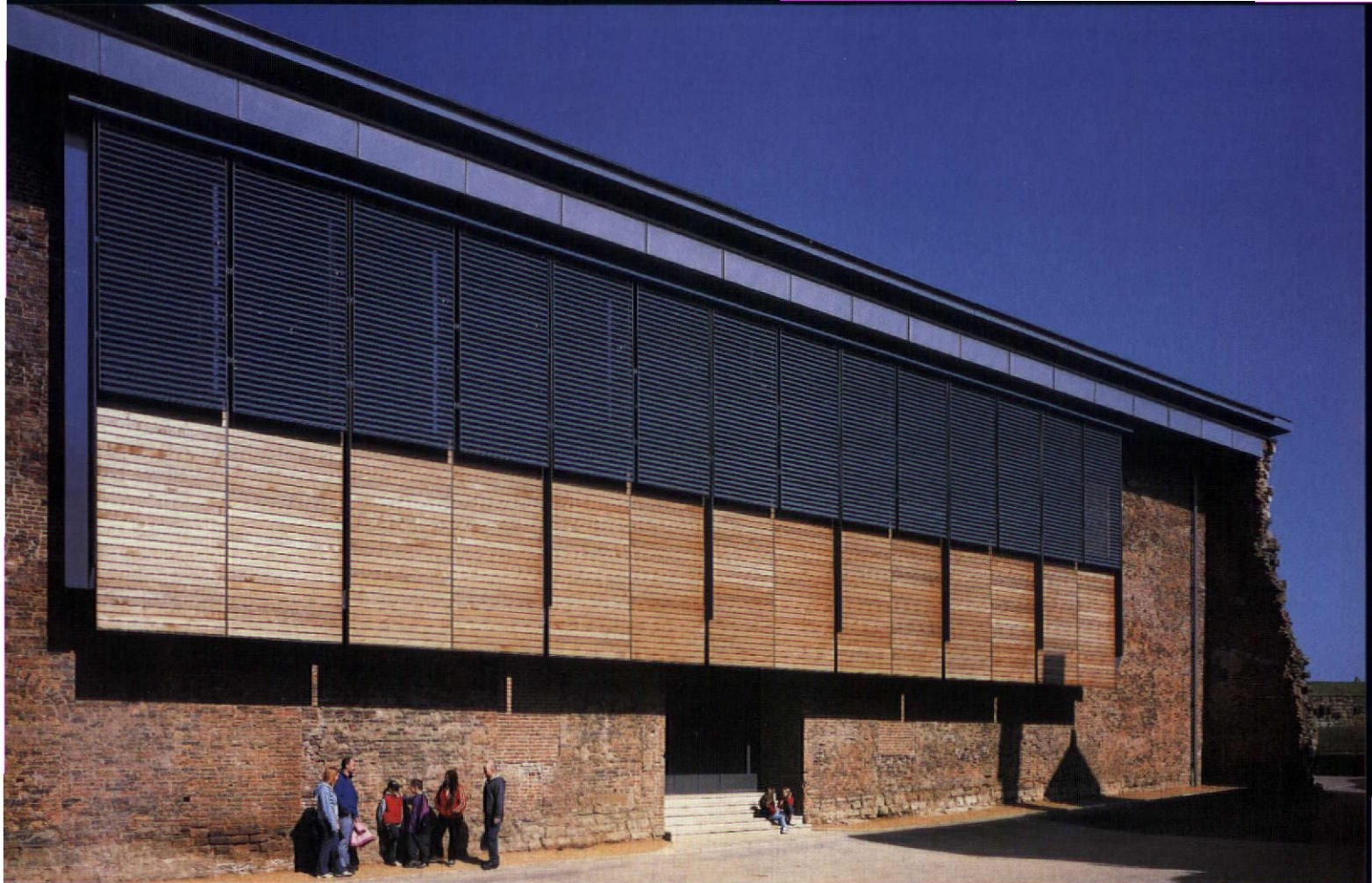
The new structure extends over the partly demolished south elevation to provide a framework from which an enclosing curtain of glass and cedar is hung
