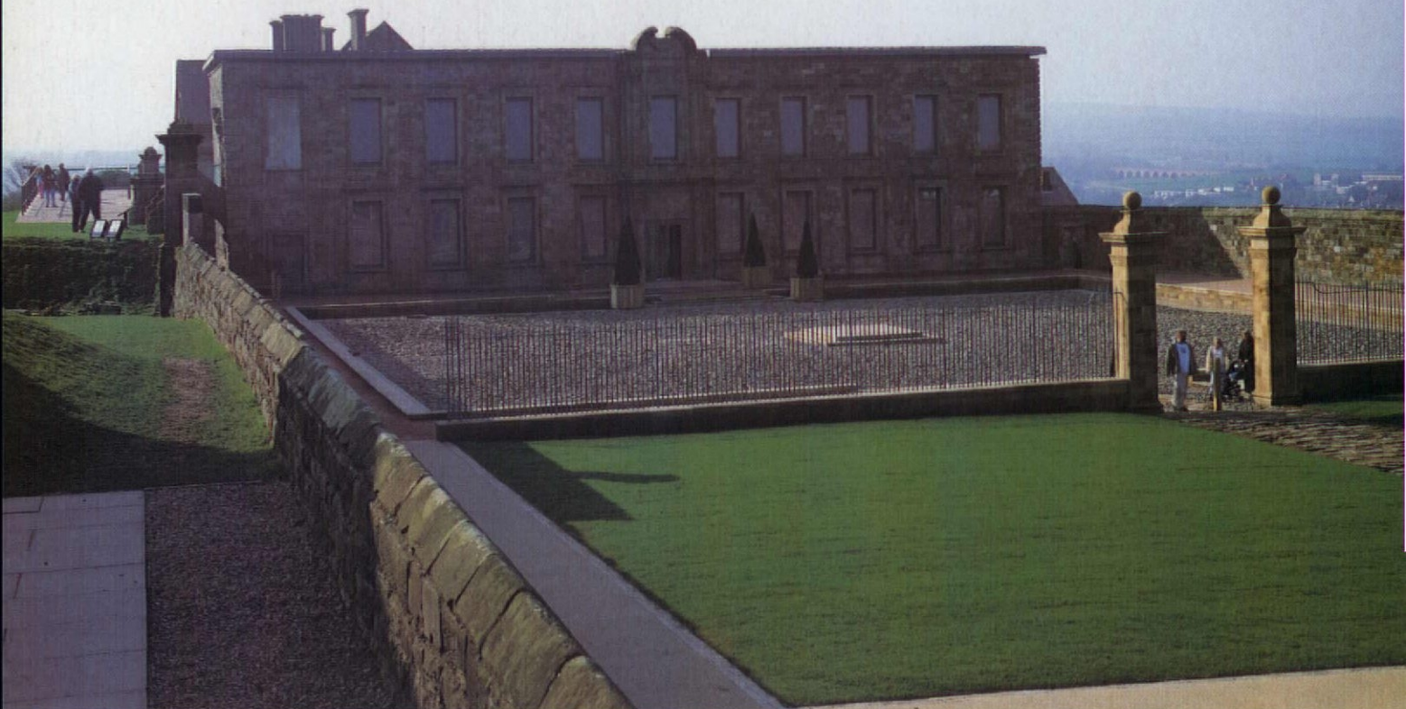
The north facade. Previously infilled windows were fitted with a single sheet of glass. Historical reconstruction was the chosen approach for the courtyards
