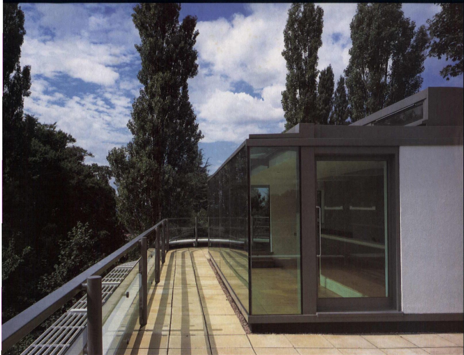
With a sun-scoop clerestory above, the lantern is detailed as a frameless glass case 'hovering' over its own terrace
