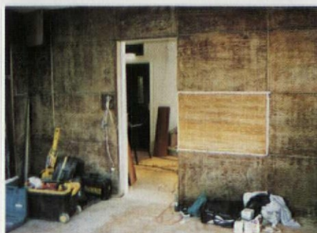
Top: Hill House before Avanti's involvement. Above: trial cleaning of timber panel in saloon
