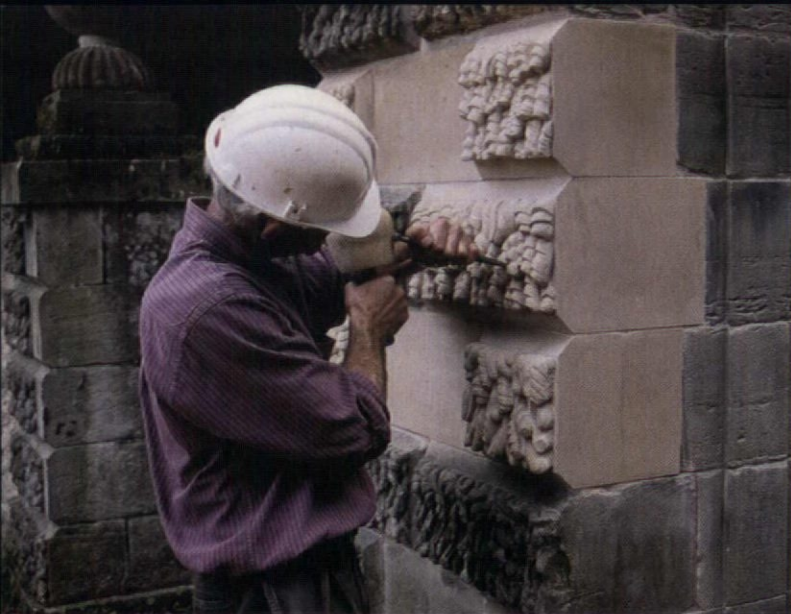
Above: new carving on the gate piers of the forecourt, being carried out by Duncan Strachan. Above right: Alex Hyland repairing plasterwork on the south elevation. Right: plasterwork on completion of repairs (white areas either side of the lichens). Opposite page: the main staircase on the south front of the house in the process of being stabilised and repaired. Only structural, not decorative, elements were replaced, and the balustrades have not been repainted
