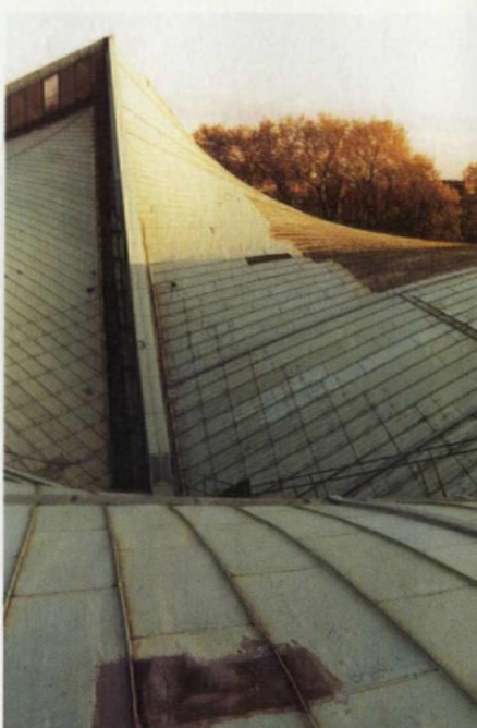
Original model for the structure, showing the complex geometry of the copper roof. Right: felt patch repairs had taken their toll
