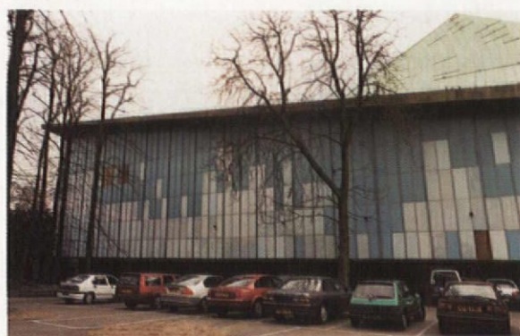
Above: the listed Commonwealth Institute with its patched-up glazing. Top: the entire cladding layer has been replaced with a new, improved reflective surface
