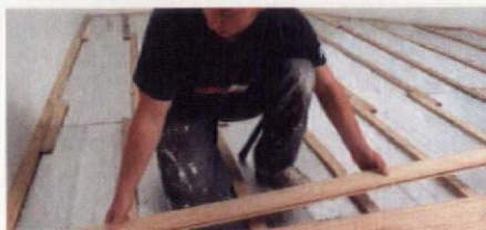
Above: installation of rigid polyurethane floor insulation. Left: thermal image showing continuity of insulation on a rigid polyurethane insulated composite wall panel
