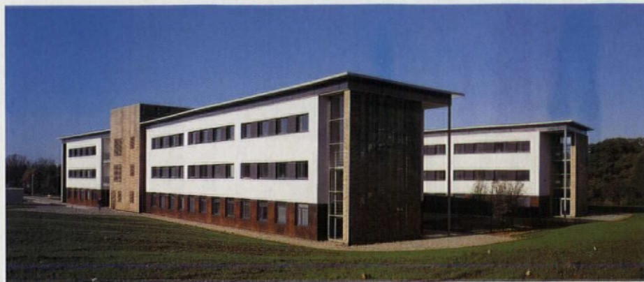
Looking west: the splayed H-shaped plan produces a high level of daylight access
